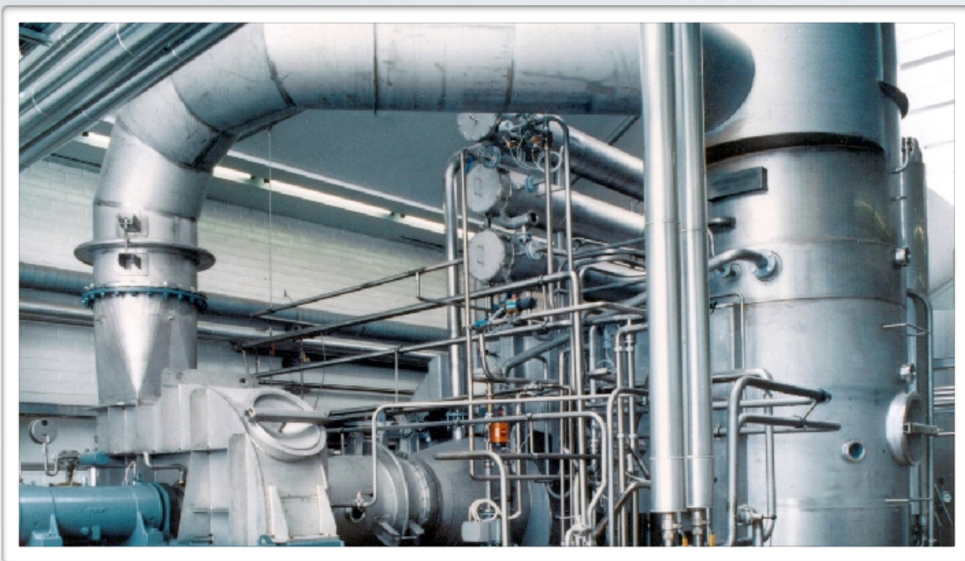
A robust industrial water recycling system has a vast market outside of the fracking industry.
