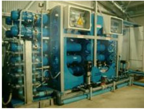
**Figure 3. Initial RO plant skid showing close-coupled motors on each pressure vessel.**
