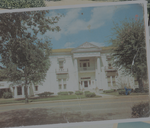
Administration Building, Lebanon, Tenn.
