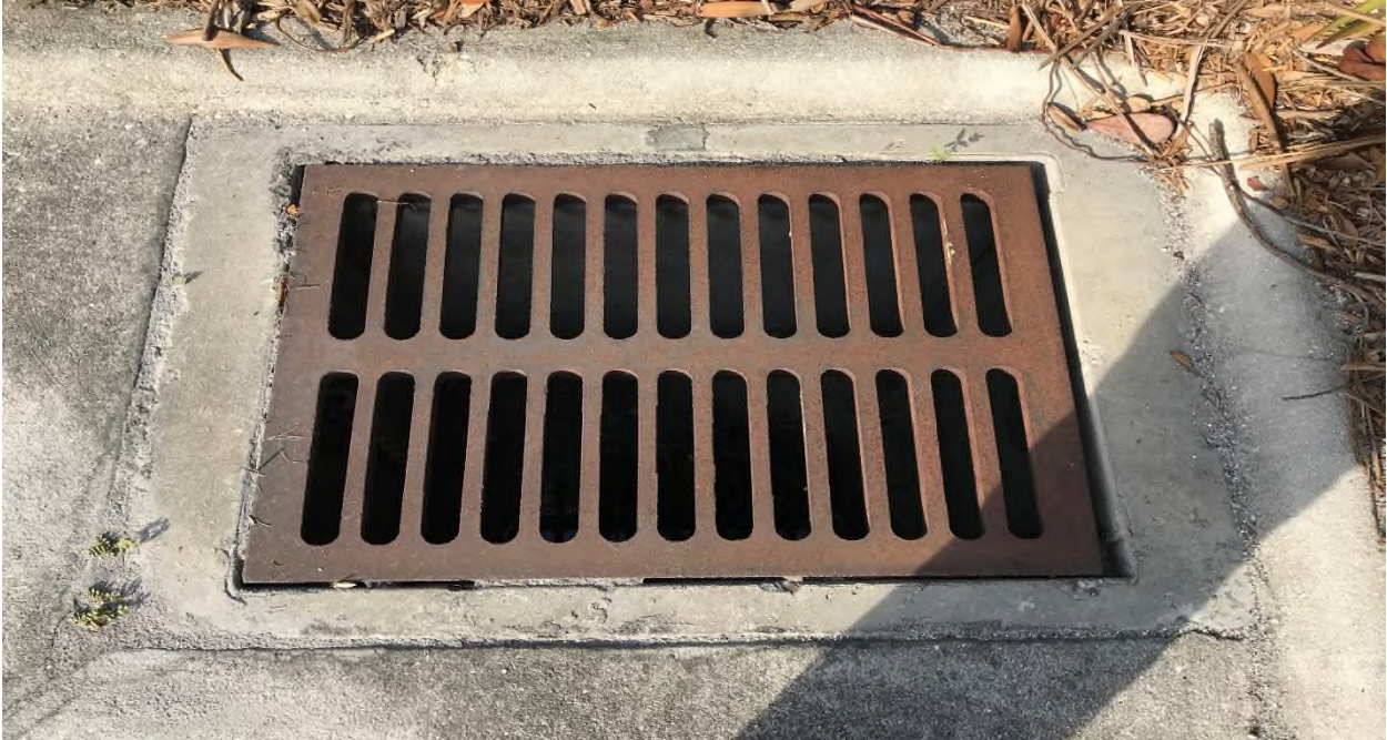
Figure 47 - Storm Drainage Inlet
