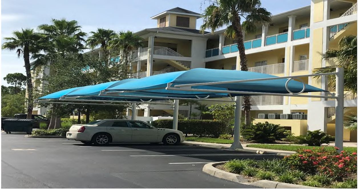
Figure 43 - Carports within Cape Haze Resort (Typical)
