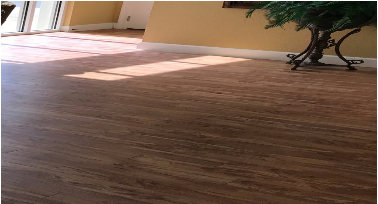
Figure 14 - Clubhouse Flooring Finish
