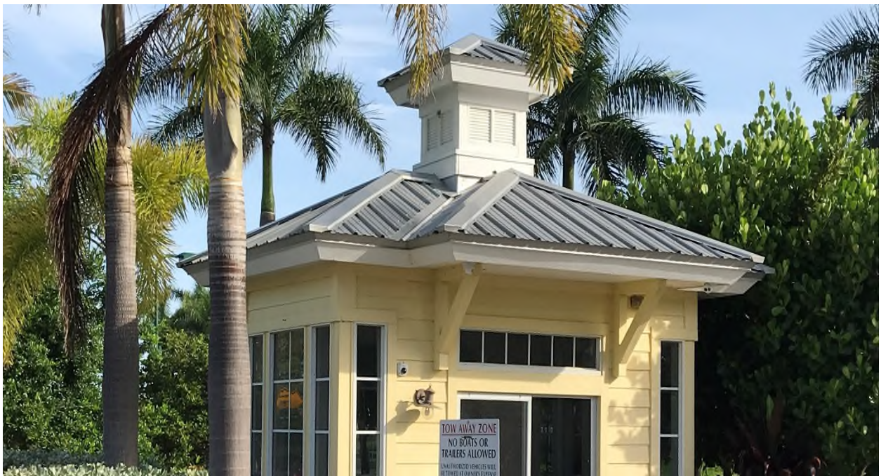
Figure 2 - Guardhouse Roofing Finish
