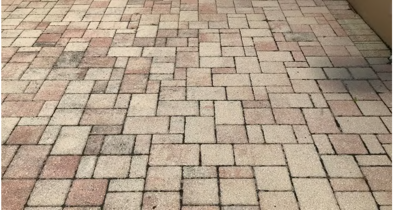
Figure 29 - Pool Patio Pavers
