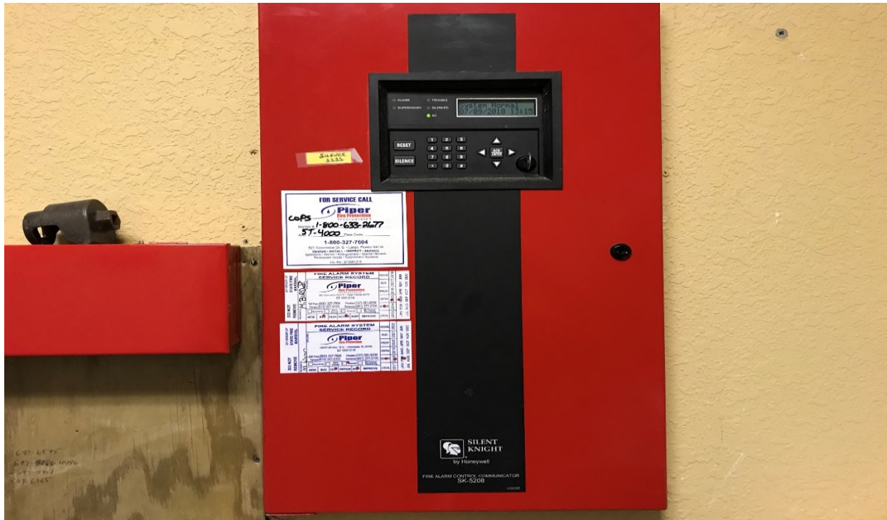
Figure 9 - Fire Alarm Control Panel
