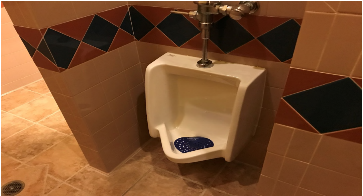
Figure 13 - Additional Restroom Fixtures
