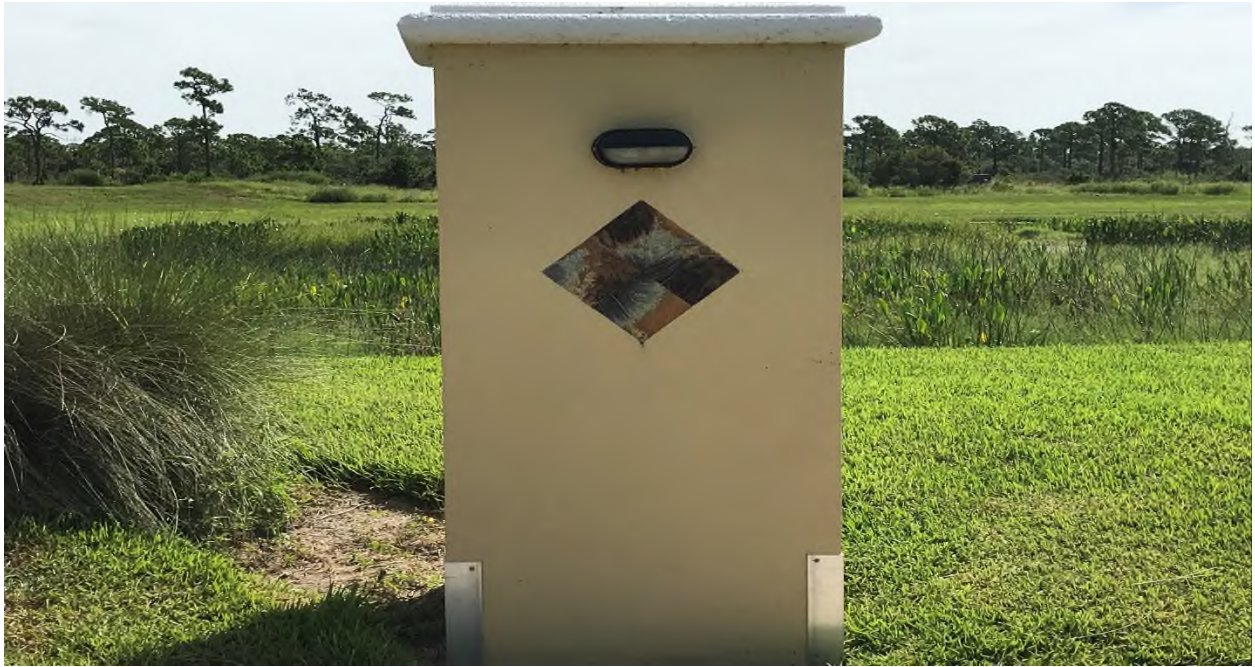
Figure 53 -CMU Perimeter Columns
