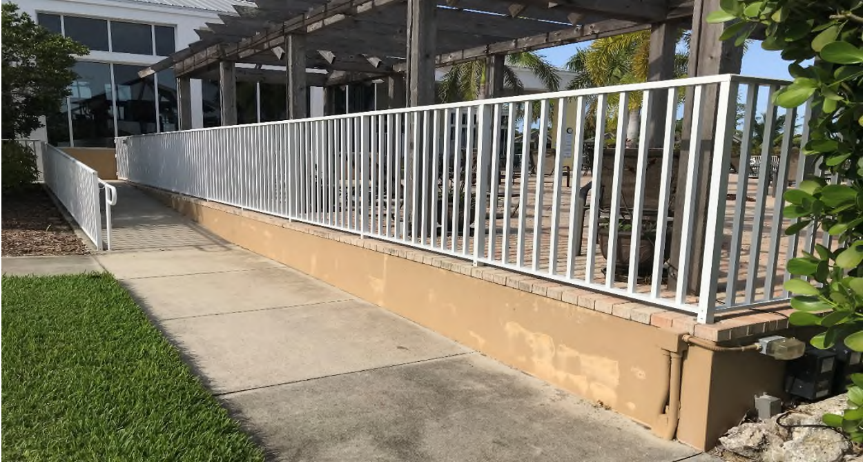
Figure 35 - Alternate View of Pool-side Railing
