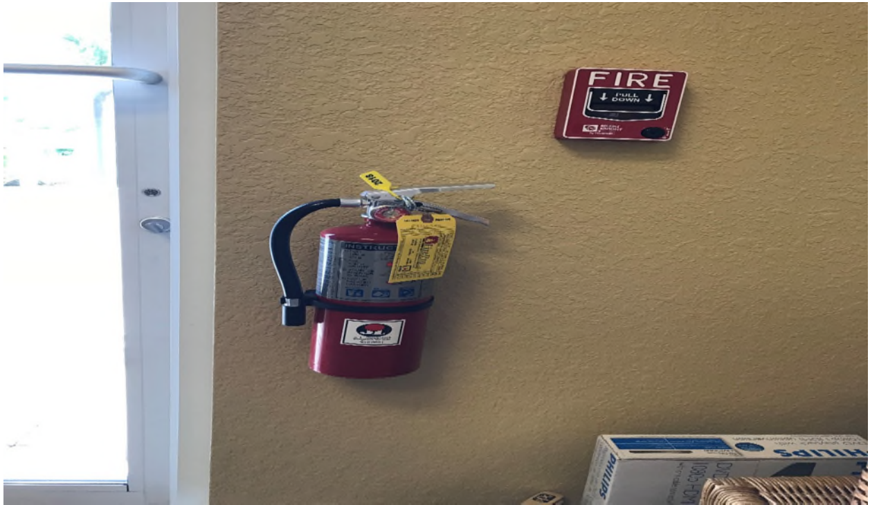
Figure 11 - Fire Pull Station & Fire Extinguisher
