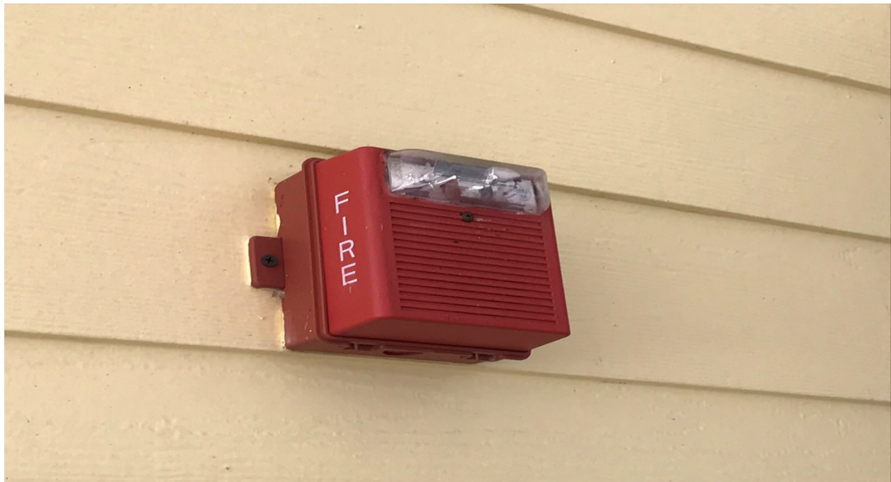
Figure 10 - Fire Alarm Strobe
