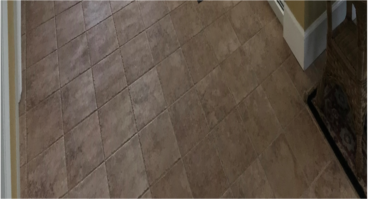
Figure 15 - Clubhouse Flooring Finish - Tile
