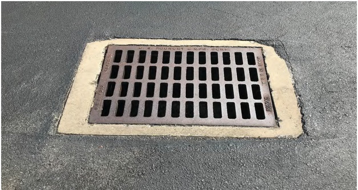
Figure 46 - Storm Drainage Inlet
