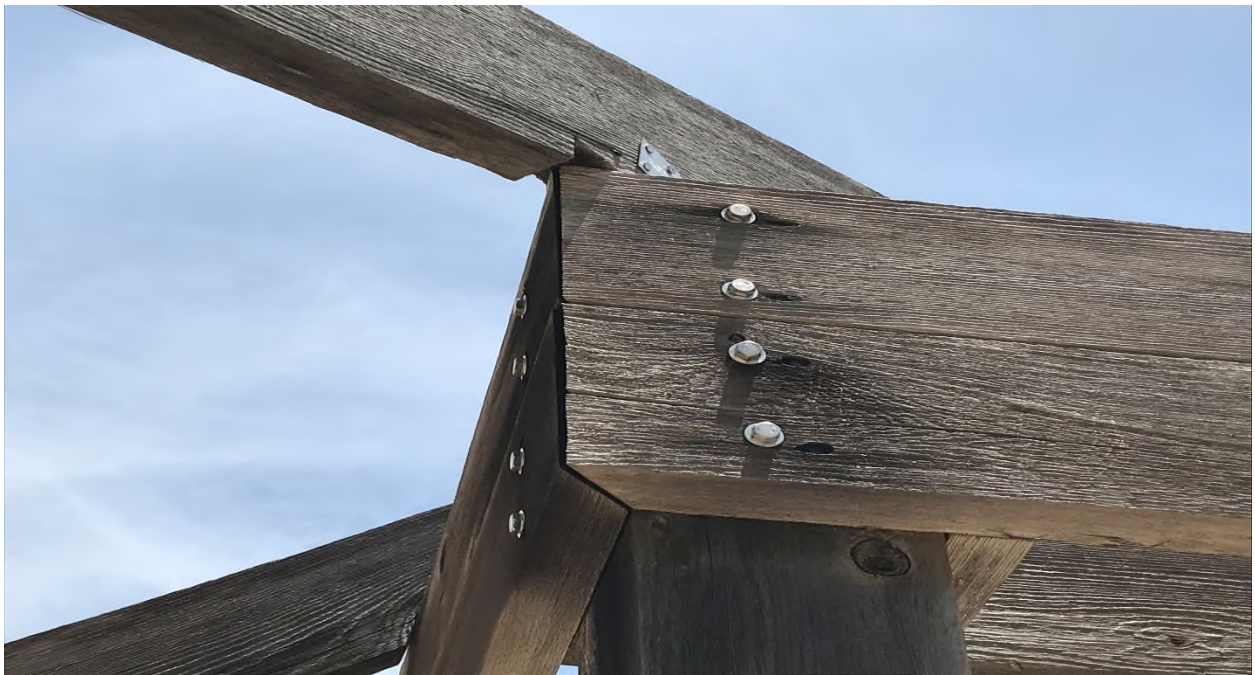
Figure 28 - Pergola Fastener Condition (Typical)
