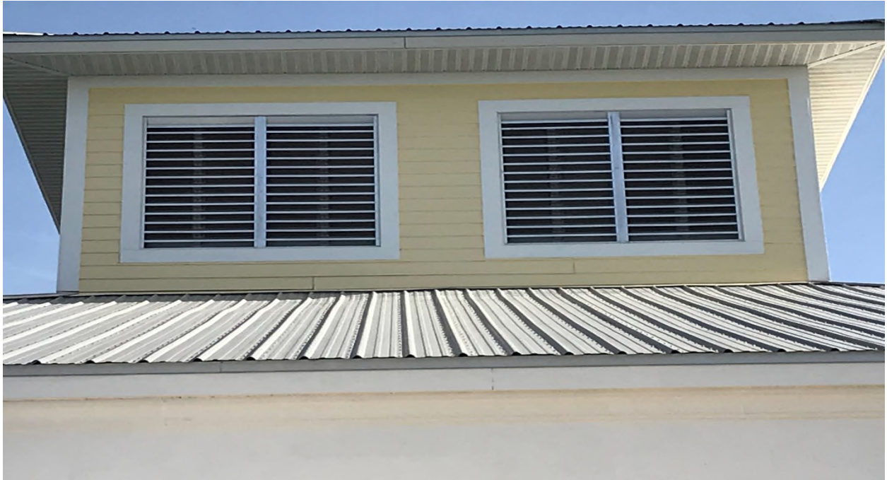
Figure 1 - Clubhouse Roofing Finish
