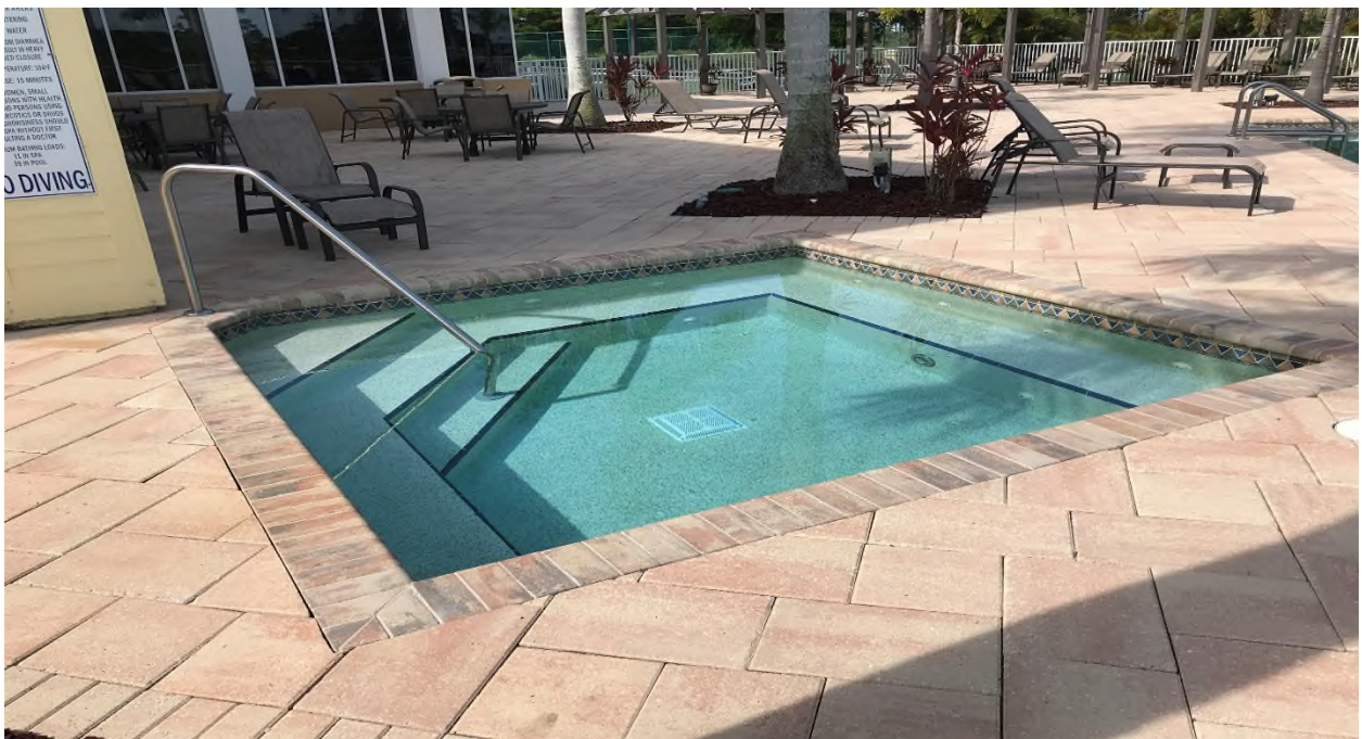
Figure 22 - Spa Interior Finish
