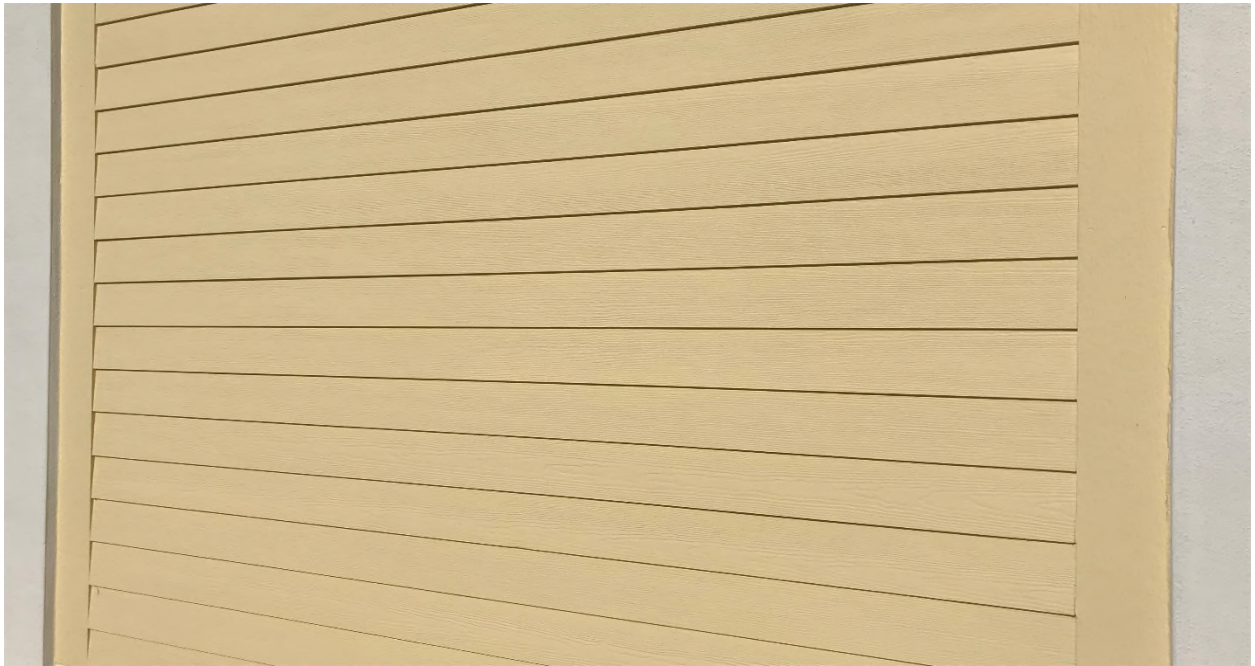
Figure 38 - Clubhouse Exterior Painting
