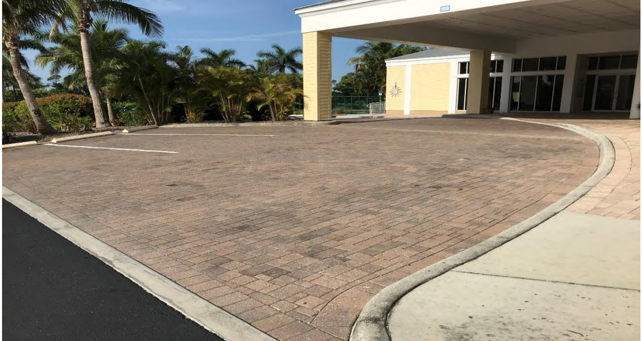
Figure 39 - Clubhouse Entrance Pavers
