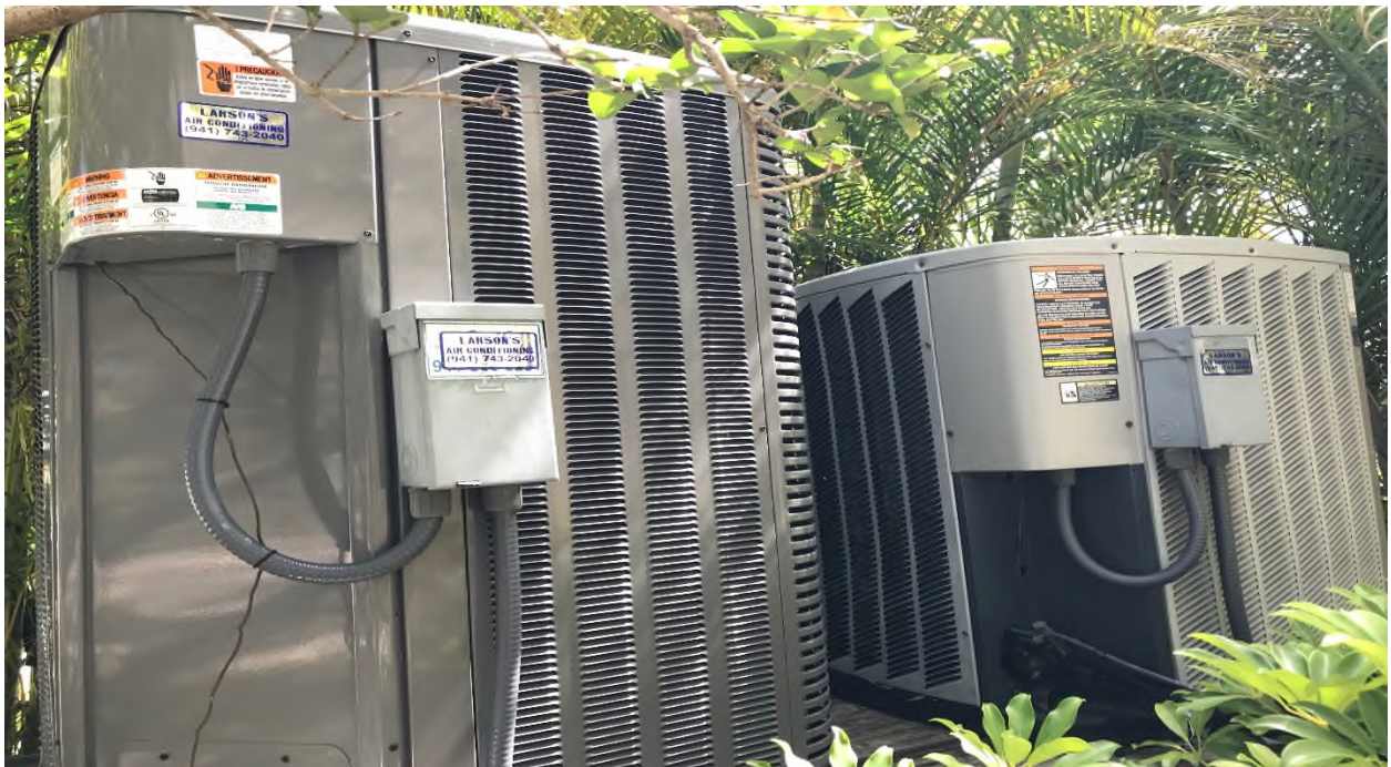
Figure 8 - Office Side A/C Condensers
