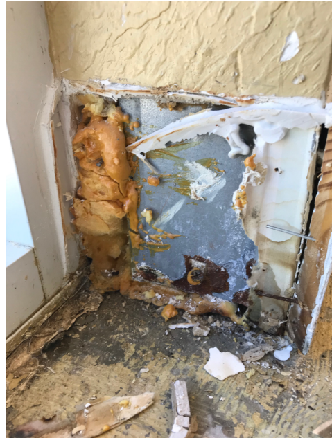
Figure 2: Board disintegration behind baseboards because of water entry at the corners
