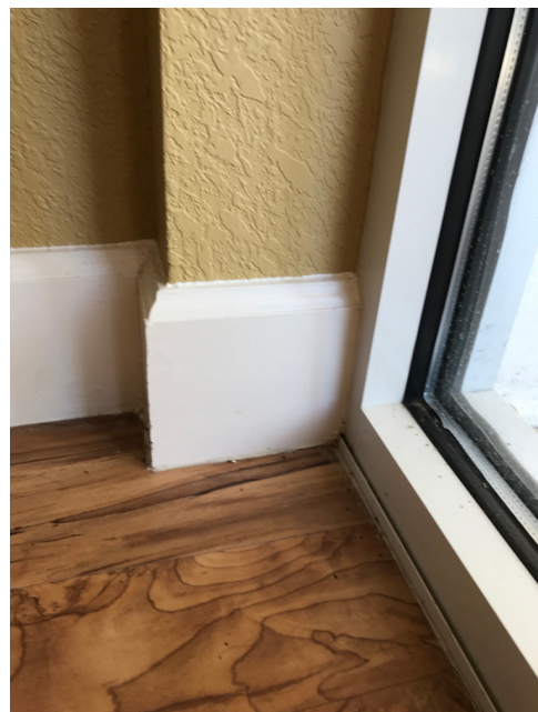
Figure 5: Wall end run under overhang which remains intact to visual inspection
