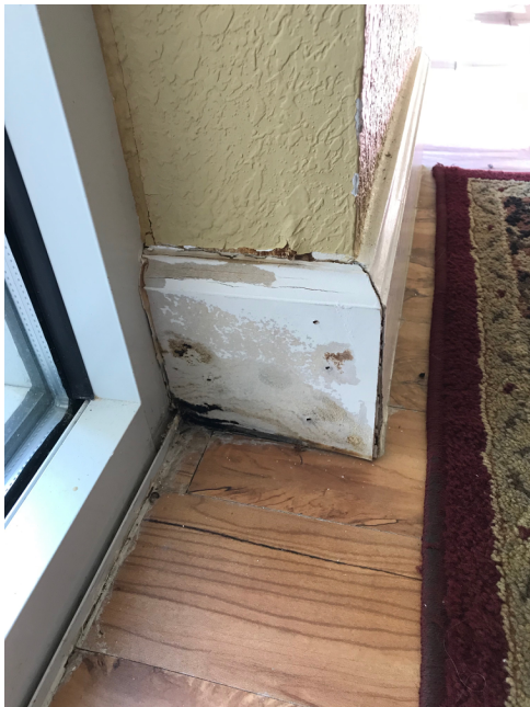
Figure 4: Wall end runs which will need to be refinished after sealing
