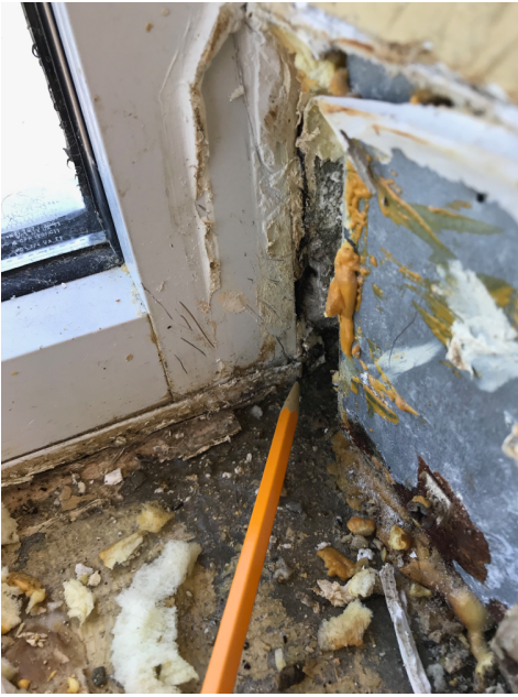
Figure 1: Water intrusion AFTER recalking sill/pan fasteners
