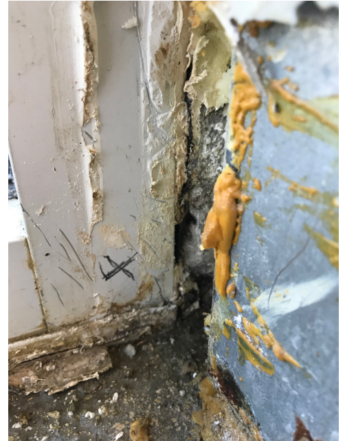
Figure 3: X marks an access hole through which sealant could be pumped to solve intrusion problem
