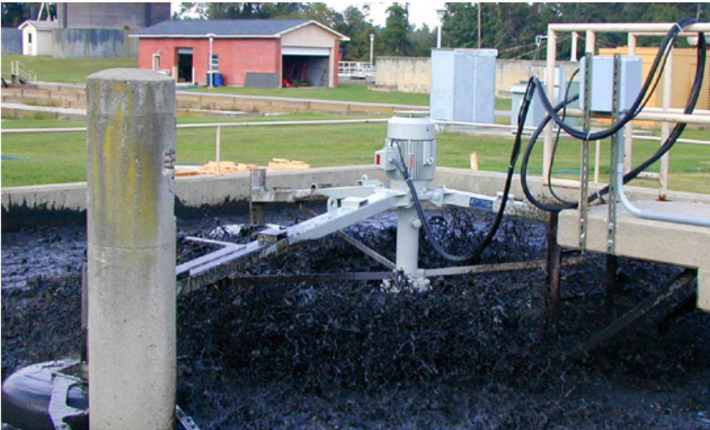
DBS Floating Aerators are ideal for lagoon and aerobic digester applications. The compact design of the NSA floating aerator makes these units easy to assemble and install. All wetted parts such as the aeration rotor, float arm lower link, and float hardware are made from corrosion resistant stainless steel for long life and reliability.
