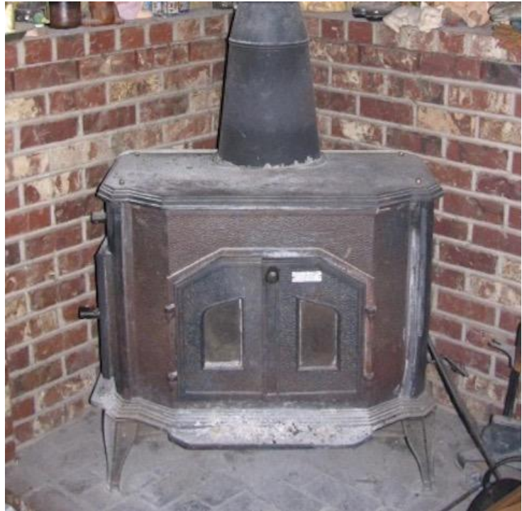
Figure 4. Example of an uncertified, outdated wood stove.
