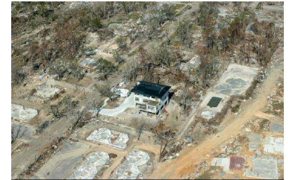
ICF House after Katrina 2005 - PCA
