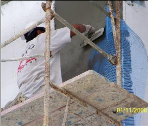
Hand applied layers and curing periods
