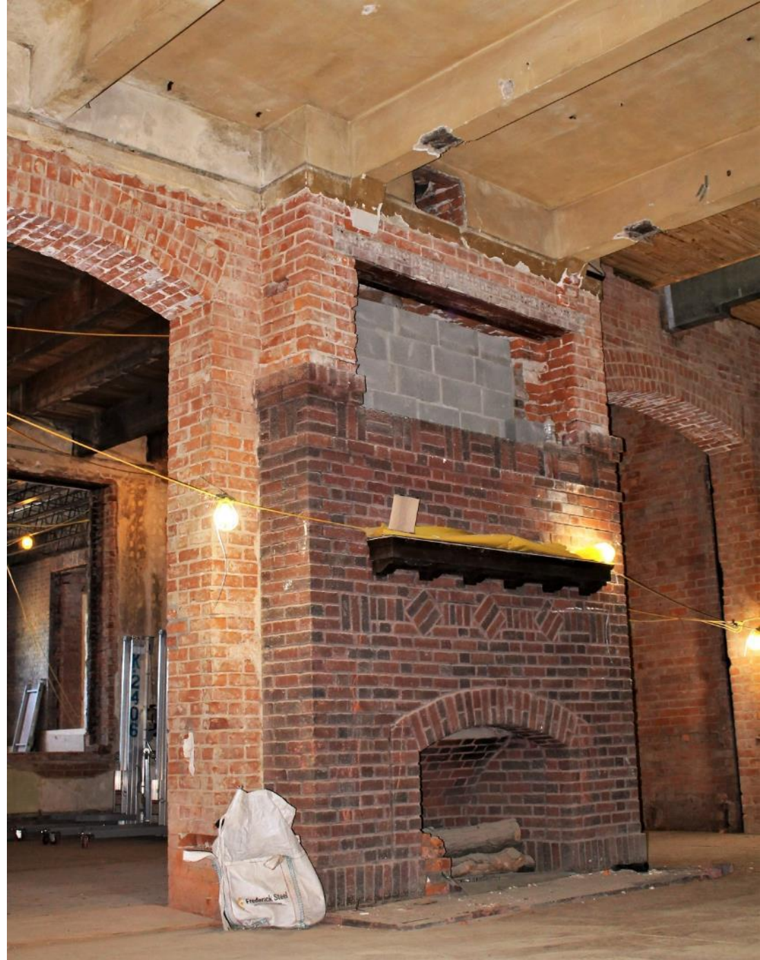
DURING CONSTRUCTION – BRICK RESTORATION
