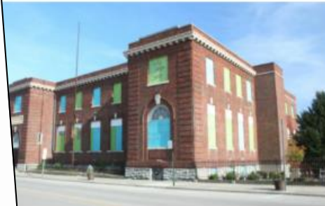
View of Office Building on Williams Avenue, looking northeast
