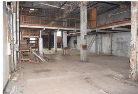
113: First-floor warehouse of 12 E. Main Street, looking southwest.
