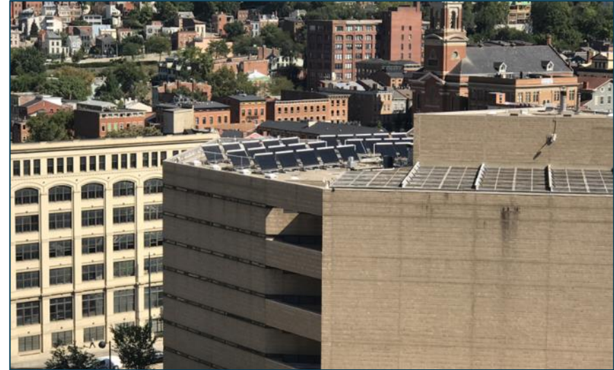
SOLAR THERMAL PANELS AT THE JUSTICE CENTER
