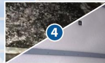
Insulation After PURE-Cell
