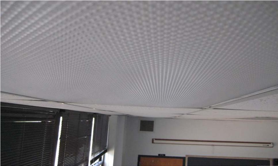
– Moisture being pulled into the building was bowing the ceiling tiles
