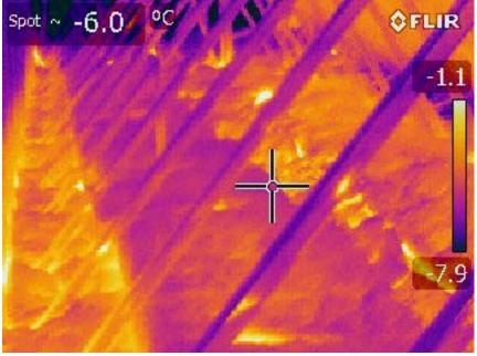
Knee wall attic, many holes in roof deck below attic space. Condensation issues
