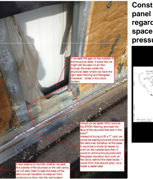
Construction: Exterior Insulated metal wal panel with Steel structural framing with no regard to conditioned & non conditioned space with significant Air leakage and pressure.
