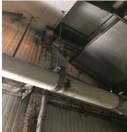
Mold / Mildew Conditioned space Metal building in humid climate
