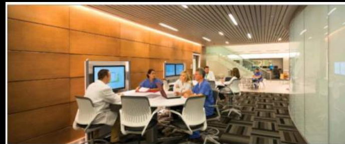
Flexible lighting fixtures at the Kaleida Health Cabot Vascular Institute in Buffalo, New York, are illuminated by BIOS lighting. Health care facilities are among the business sectors in which BIOS believes its lighting technology will find traction.
