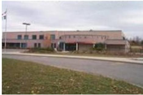
This school is constructed with conventional brick / masonry construction. It took 8½ months to construct.
