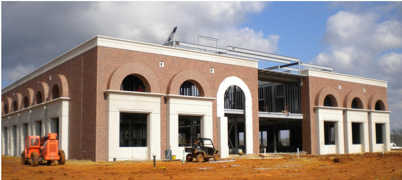
***Tilt-Up Concrete complies with section C402.4.1.2.1
