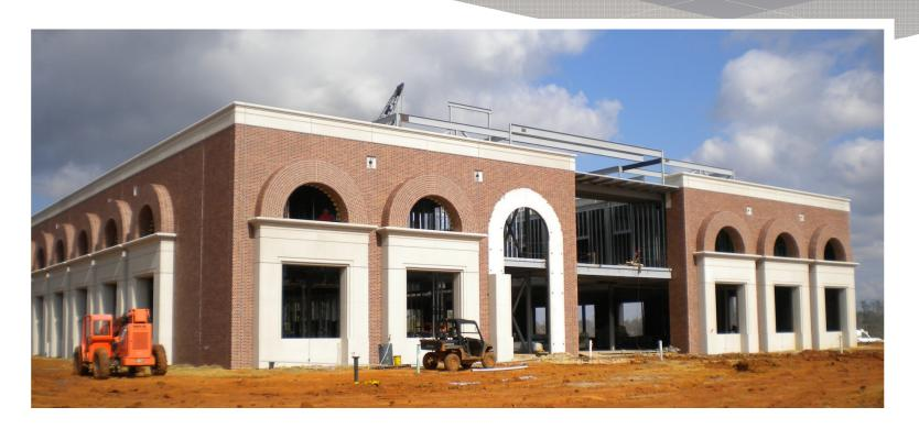
Tilt-Up Concrete complies with section C402.4.1.2.1 with air permeability of 0.004 cfm/ft2 or less
