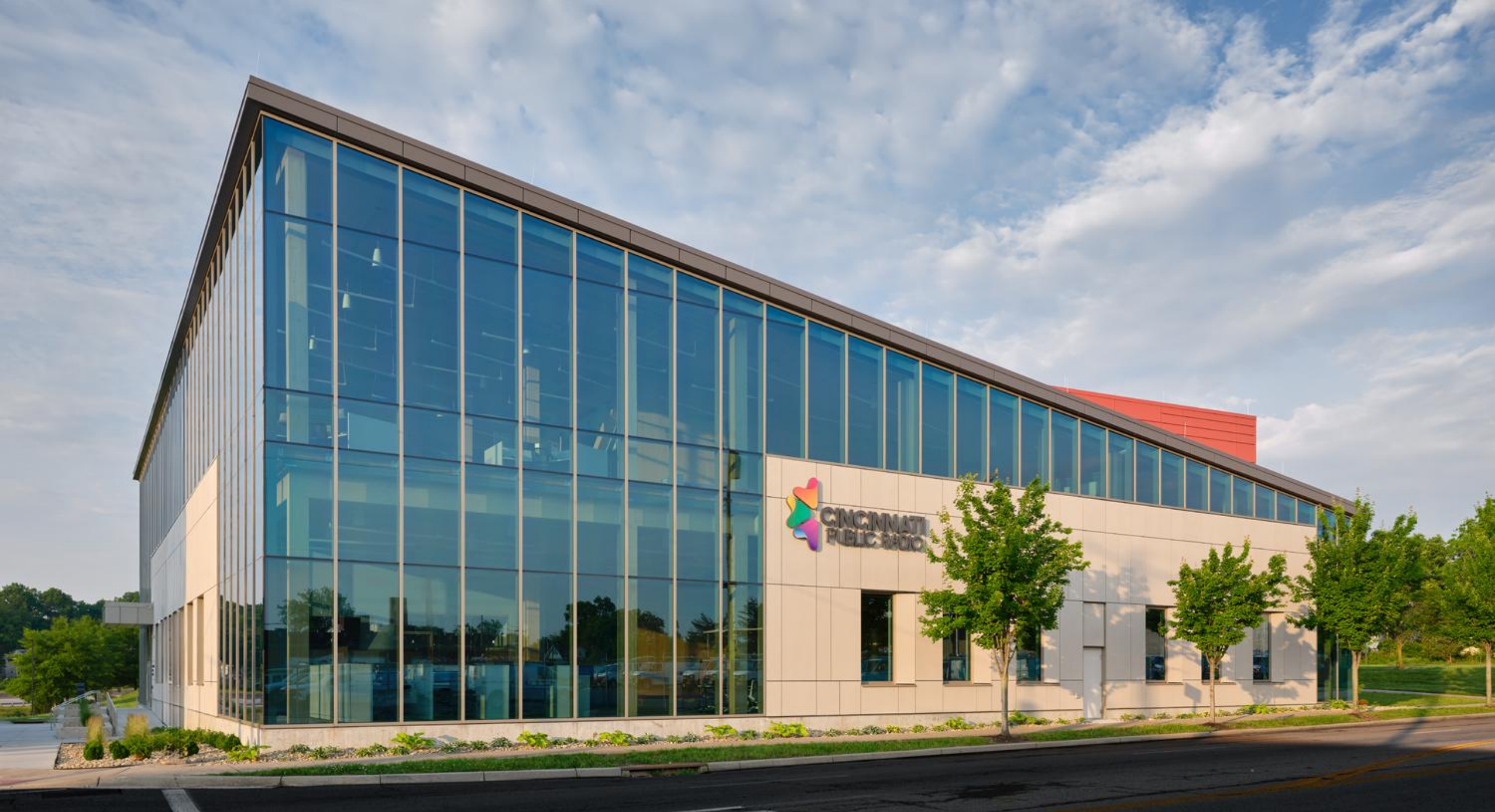
Exterior – North view
