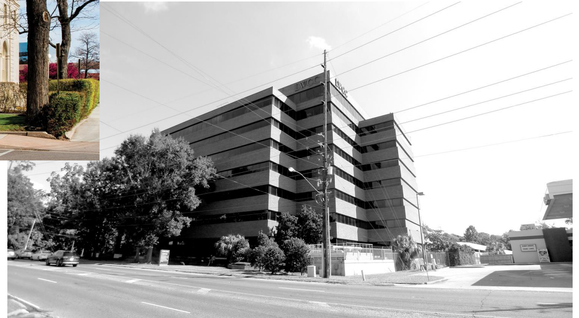
LWCC HEADQUARTERS (1984, 2020) BATON ROUGE, LA | EUI 96→27 ESKEW DUMEZ RIPPLE
