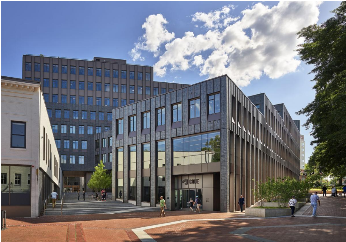
Center of Developing Entrepreneurs (CODE) | Charlottesville, VA | 2022
