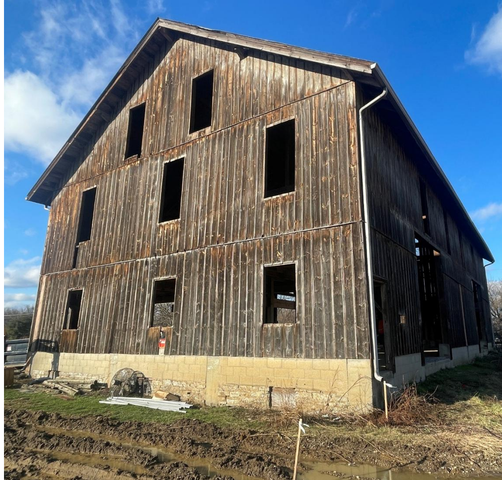
Demolition and Prep
