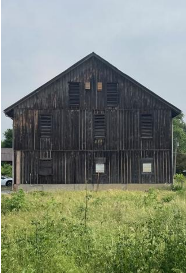
Existing Drying Barn
