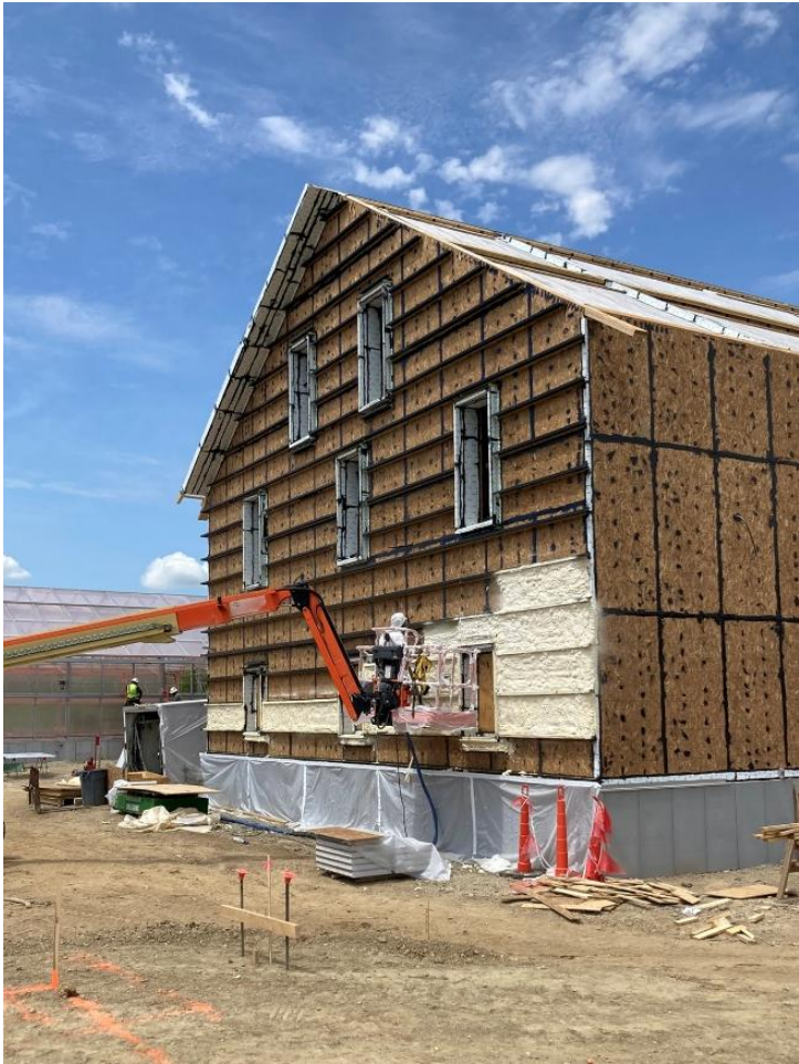
New Insulation Air/Vapor Barrier
