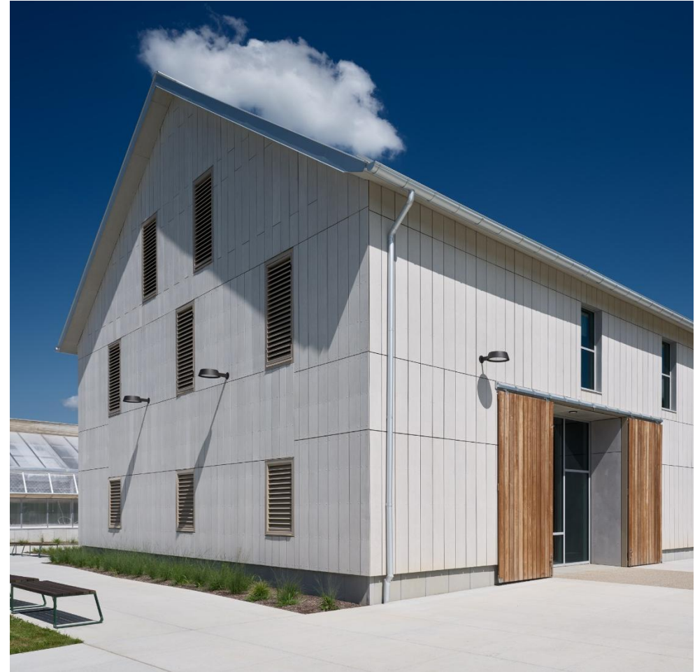
Final New Thermal Envelope And Bat Louvers
