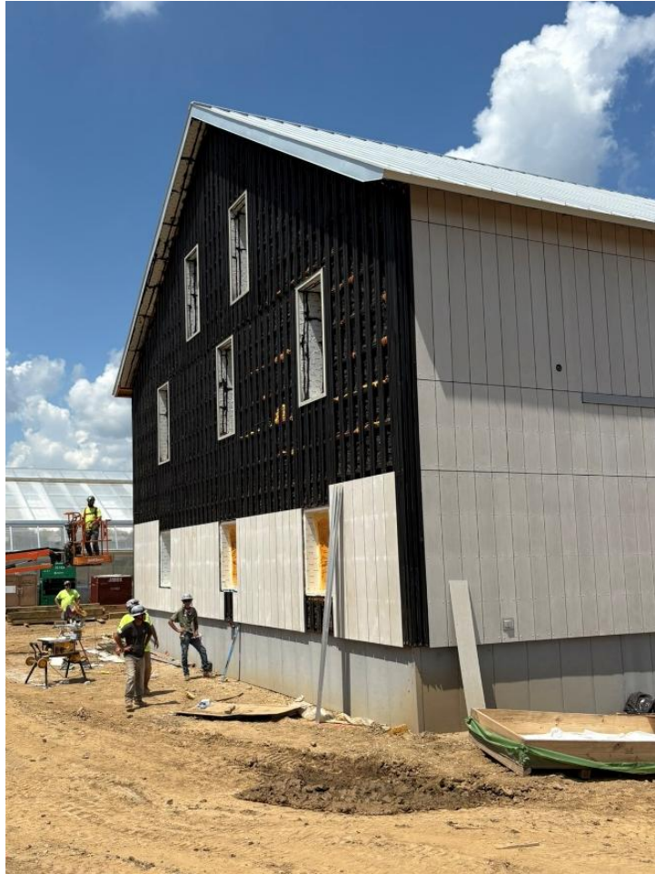
New Fiber Cement Siding And SIP Roof
