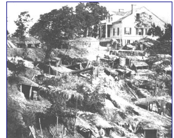
The Confederates dug bomb-proof shelters on the reverse side of their lines
