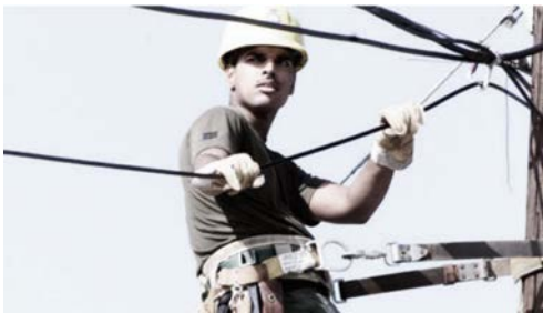
Figure A-20 Line Technician
