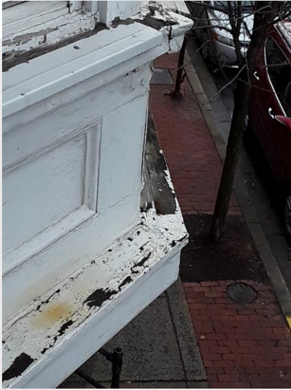
Though certainly not visible from the street, defects like this will prevent the inspection from proceeding
