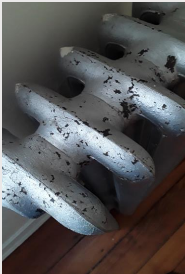
Radiators and the wall behind them are often overlooked when making paint repairs.
