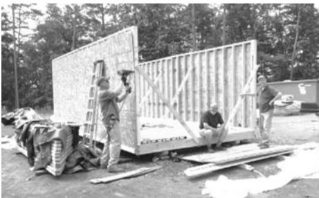
The FPC Annex (shed) under construction by the men of Faith, Hope, and Hammers. Pictured from left to right are Jim Reich and his 2 supervisors Jim “Bunns” Bunnelle, and Glenn “Spiderman” Ferris. Finished it has resulted in a great storage facility for our new church.
