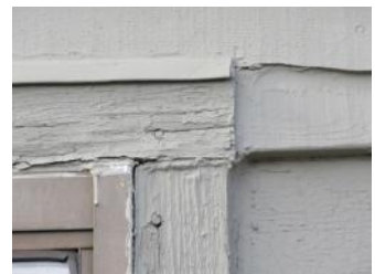
Ideally, flashing should expand past window trim.
