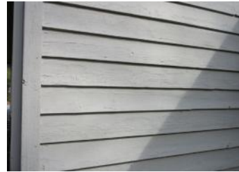
Due to the age, paint preparation could be significantly higher than in previous painting cycles.
