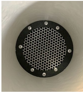
Figure 5 Protective Debris Screen inside the Litter-Vac canister.
