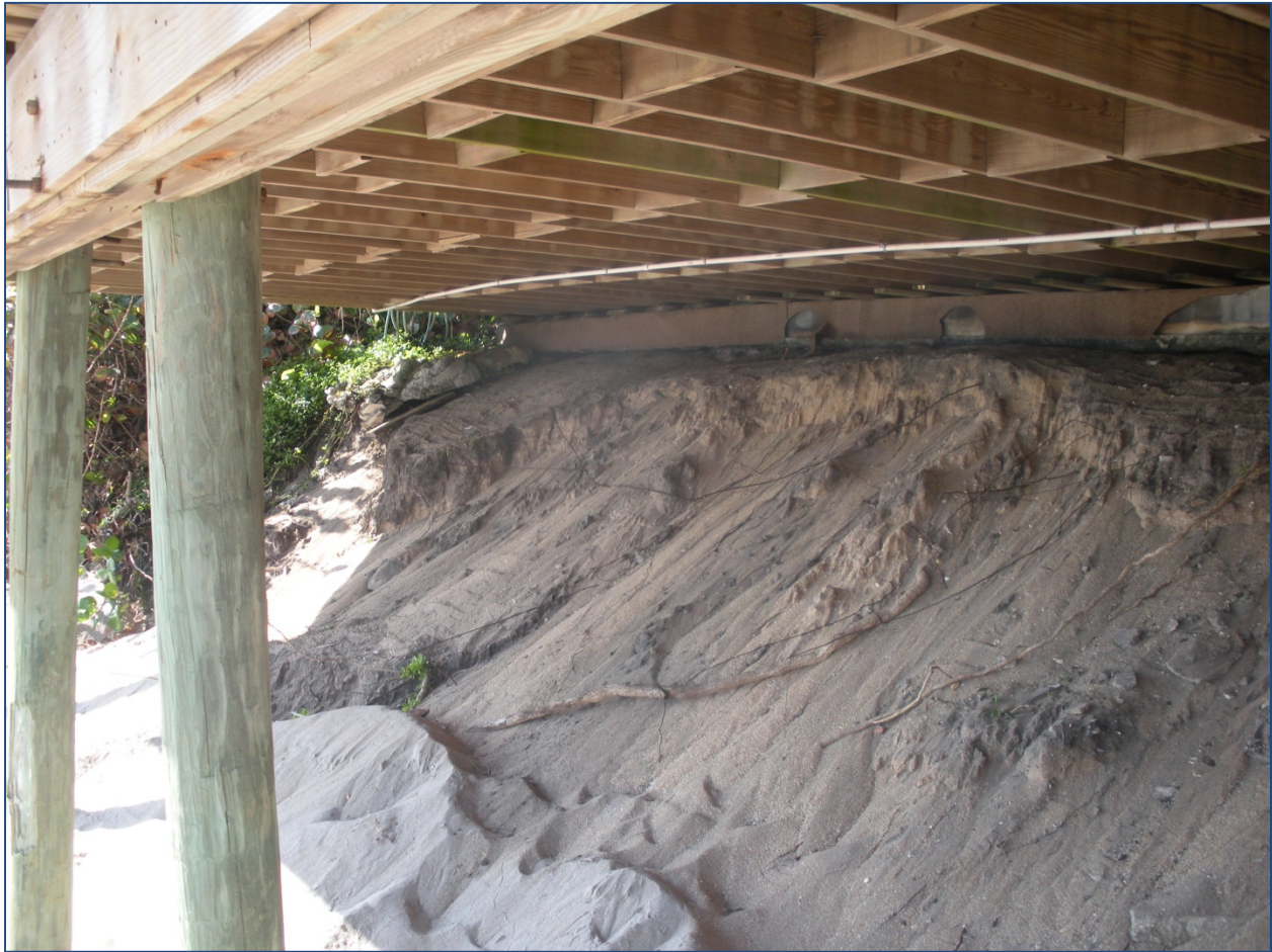
Photo 8. Deflation of the dune underneath the deck at 4513 S Ocean Blvd, likely as a result of Hurricane Sandy.
