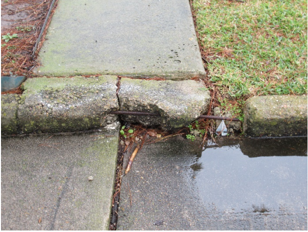
Damaged concrete and exposed reinforcement steel
