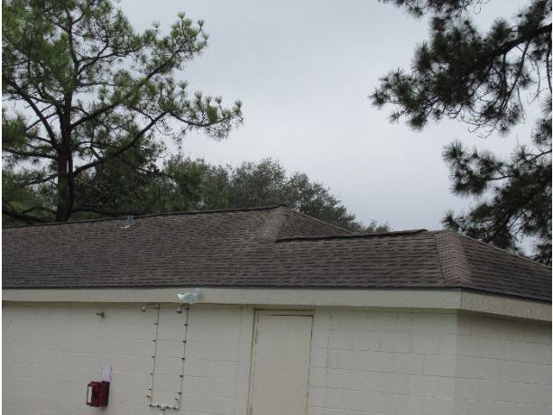
Asphalt shingle roof – Note minor discoloration
