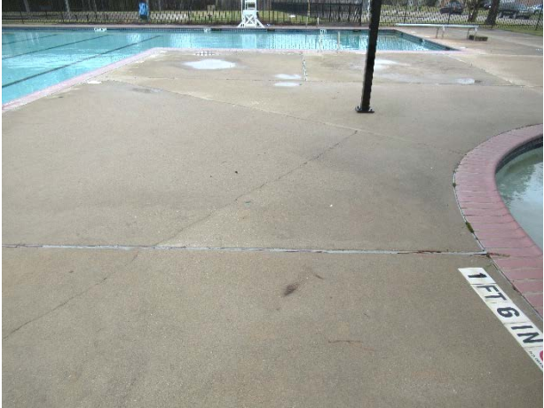
Concrete deck – Note cracks
