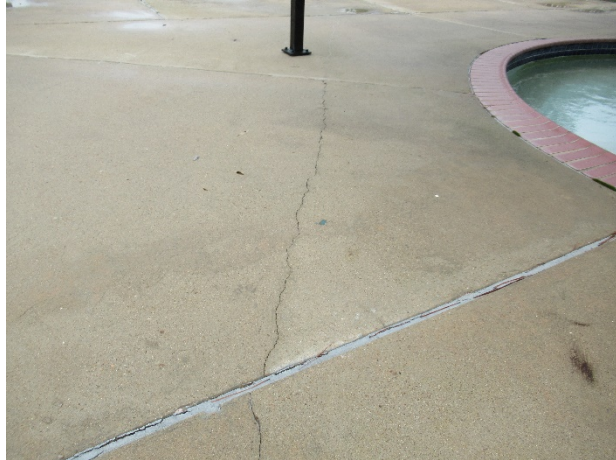
Concrete cracks
