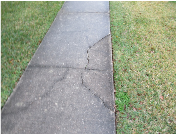
Concrete cracks
