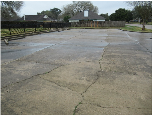
Concrete parking lot – Note cracks
