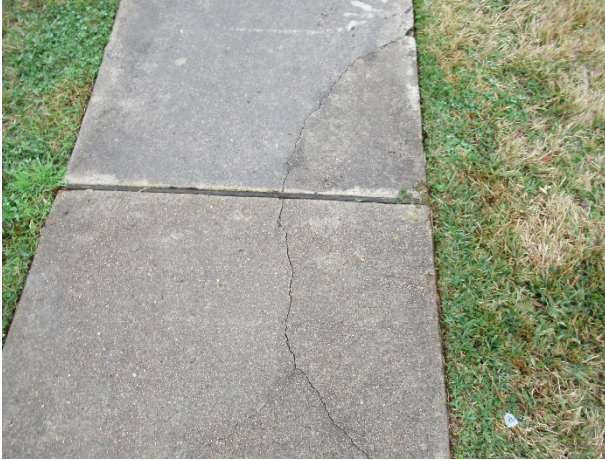
Concrete cracks
