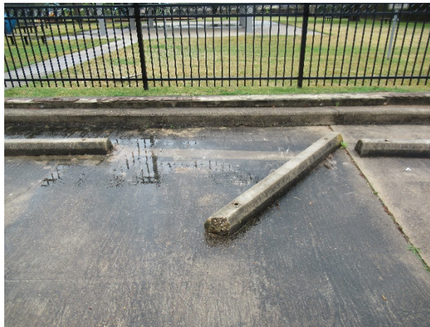
Displaced concrete wheel stop
