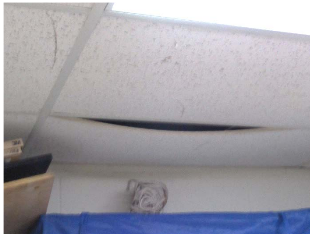
Damaged ceiling tile at the storage room
