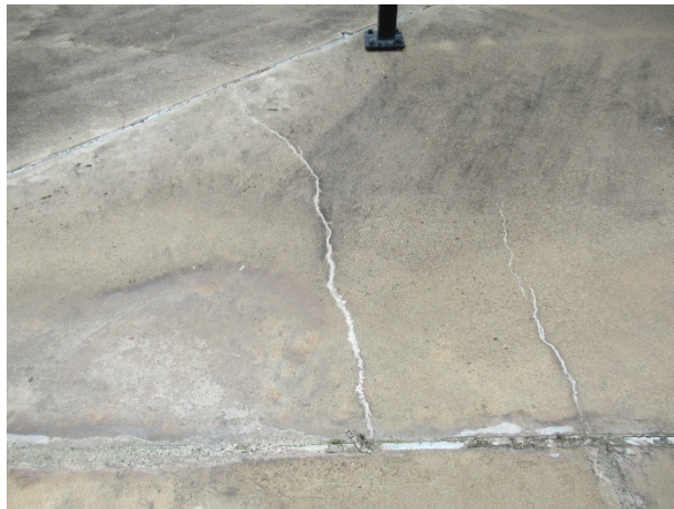
Previously repaired concrete cracks
