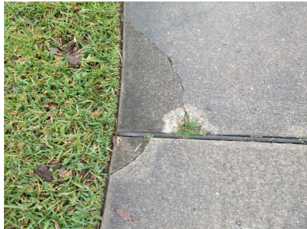
Concrete cracks and spalling
