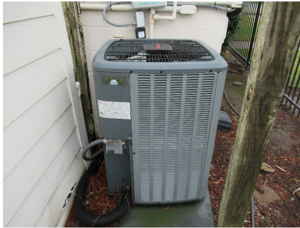
External condensing unit
