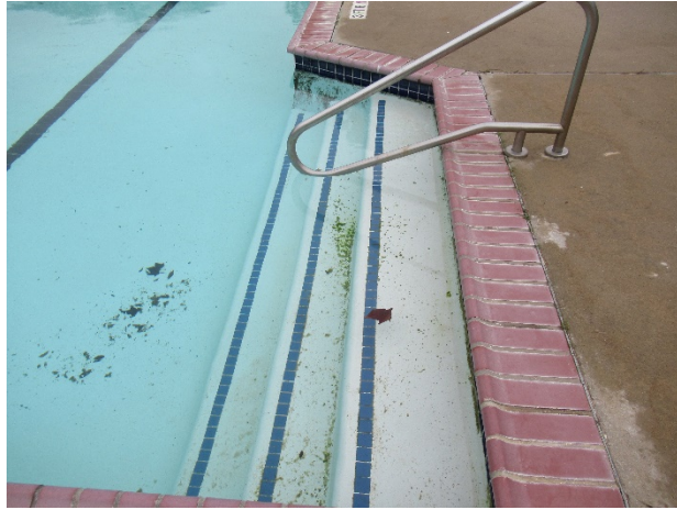
Pool plaster and tile finishes – Note algae
