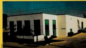
Foothill Glass Company Headquarters, Irwindale, California, was coated by Seal-Tech, Inc., with the new Dow Corning® AllGuard Elastomeric Coating. The coating provides the benefits of weatherproofing and the aesthetics of custom color.
