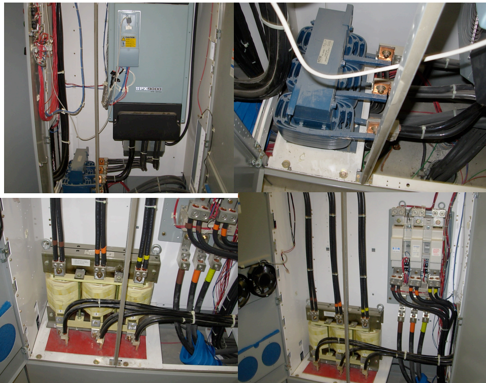
The pictures above are of the Motor control center.
