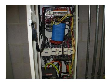
This is the VFD box after the CoolBLUE® cores and NaLA® cores were installed. This VFD controls 3 - 20hp fans motors in parallel. The Cores were installed on the top side of the contactor, the contactors on the left and the right of the center contactor are for the bypass part of the drive. We installed four - M283 CoolBLUE® cores and three - M-381 NaLA® cores.
