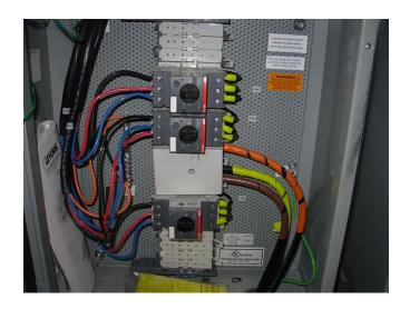
This box is the parallel connection and the overloads for the 3 motors.
