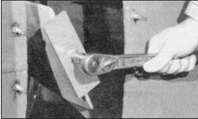
Figure 7. Adjustment of ducted inlet fans
