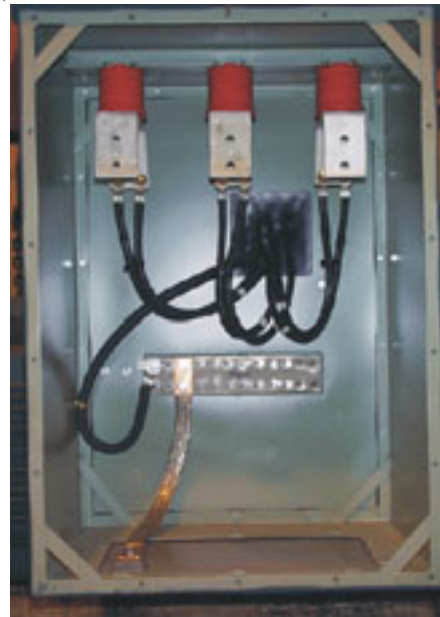
Figure 8: Ground bus connection pad in variable speed motor conduit box.
