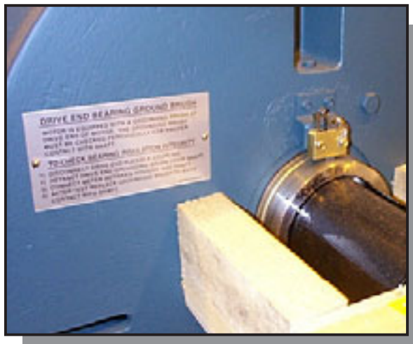
Figure 26: Shaft grounding brush.
