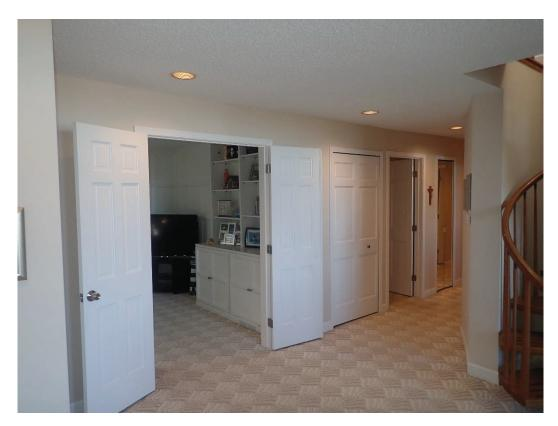
Photo #5 – Unit 3444: No gypsum board cracks in walls or wall opening in south hallway.
