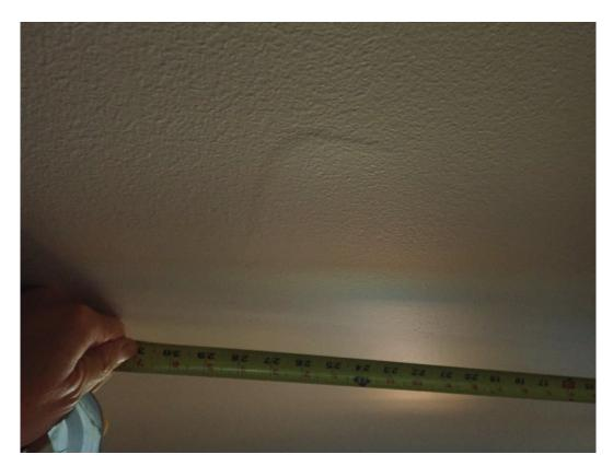
Photo #19 – Unit 3442: Bump in ceiling gypsum board finishes approximately 26" west of south post, formerly southwest corner pantry that was removed.
