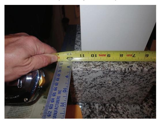
Photo #16 – Unit 3442: South post out-of-alignment with north post, 3/4" toward west.
