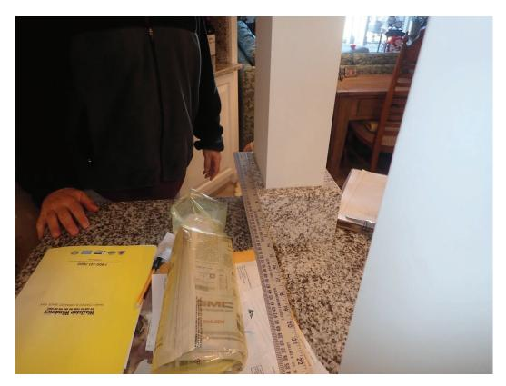
Photo #15 – Unit 3442: South post out-of-alignment with north post, 3/4" toward west.
