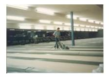
The final sanding to the lanes is done with a Progress Oscilator, using a fine grit of sand paper, followed by two screenings to close the pores of the wood. This first screening is done with a rotary and the second is done with an oscilator. The oscilatior will remove any swirl marks that a rotary might leave.
