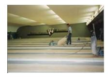
The approaches (not pictured) are also fine sanded with two different grits of sand paper, followed by a screening, using a rotary.
