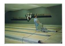
Next we remove the finish from the first few feet on the lane side of the foul line with a 12" drum sander. The Gallicchio Maxi Sander reads this as a low area, due to the approach being thicker then the lane, thus it will not sand this area. We first sand this area at a 45 degree angle to make this area flat and then we sand with the grain to remove any 45 degree marks.
