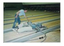
Once all of the finish has been removed and the lane is level, the bowling lane is ready to be fine sanded. We start using the Gallicchio Longitudinal Belt Sander. This usually requires a couple of passes, using two different grits of sanding belts. This sander will remove the sanding marks from the coarser paper used by the first sander. Very little wood is remove with this sander.
