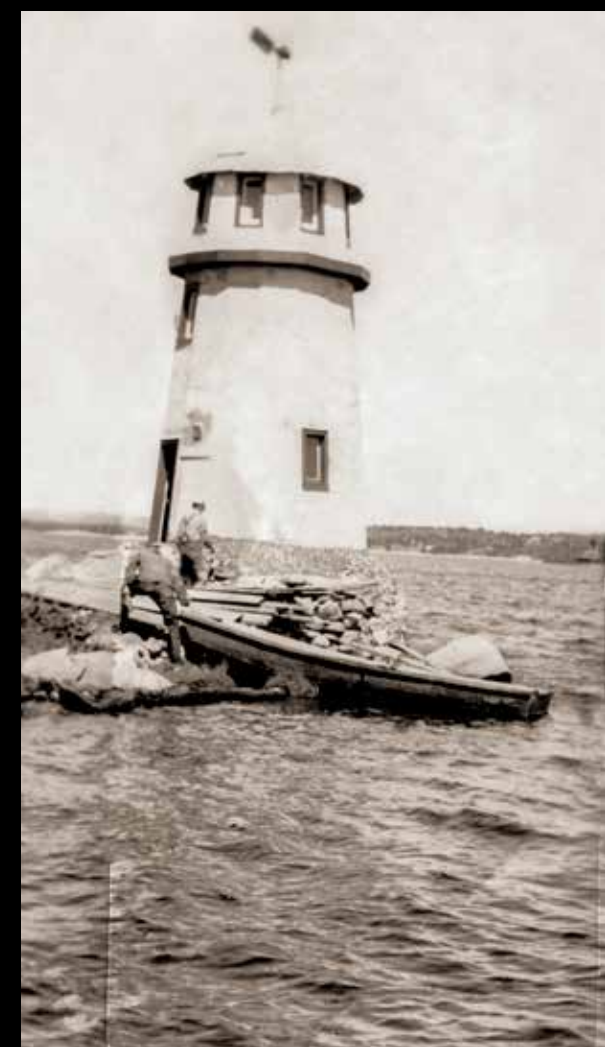
Construction of the Lighthouse.
