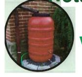
Rainwater harvesting-Rainbarrels and downspout planters can reduce stormwater runoff by holding water from roofs, which keeps polluted water from entering our creeks.
