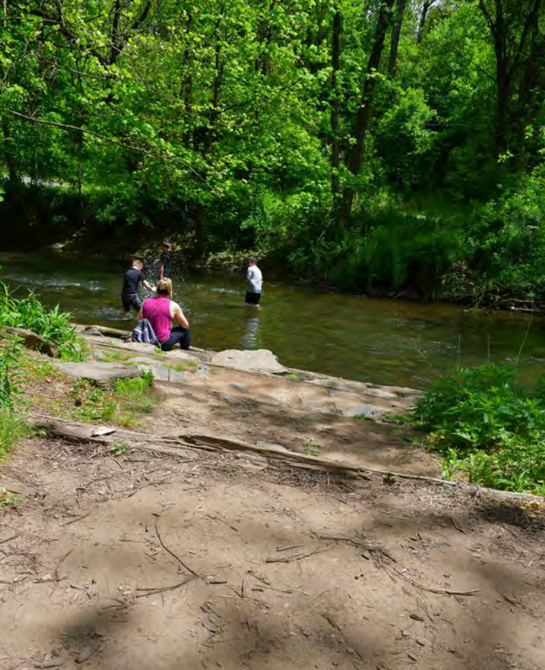
Stepped boulders can allow for informal stream access while serving to protect the banks from erosion.
