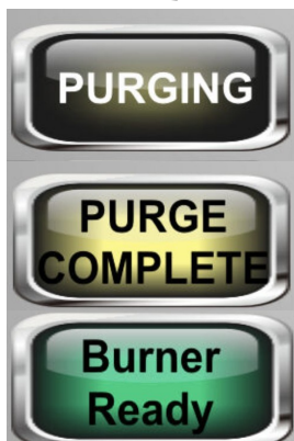
Burner Purge Status Display
