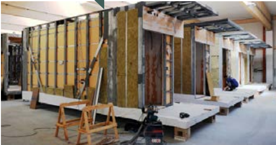
All modules are fully prepped with insulation, electrics & A/C units
