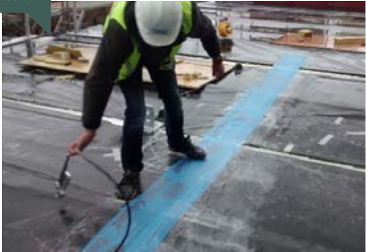
Joints between modules are sealed
