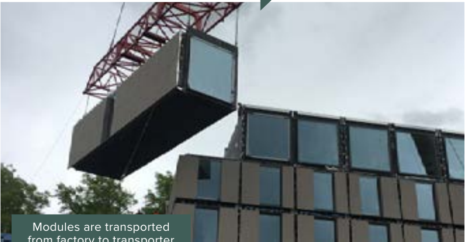
Modules are lifted into position by crane
