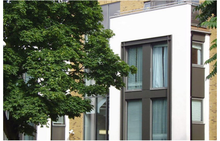
Fig.2 Modular housing with partial brick facade, London
