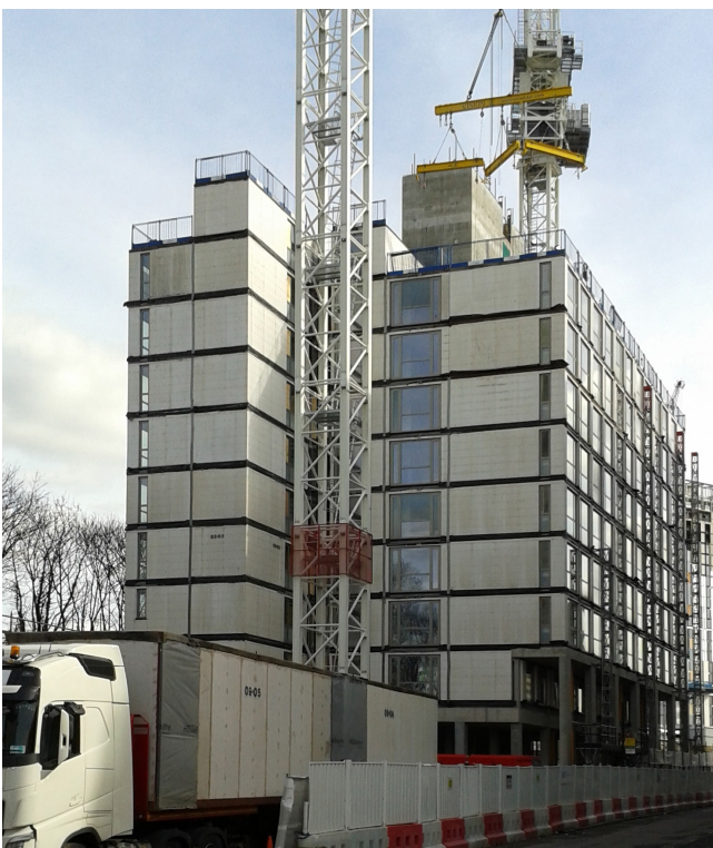
Fig.7 Modular installation in Lewisham, London
