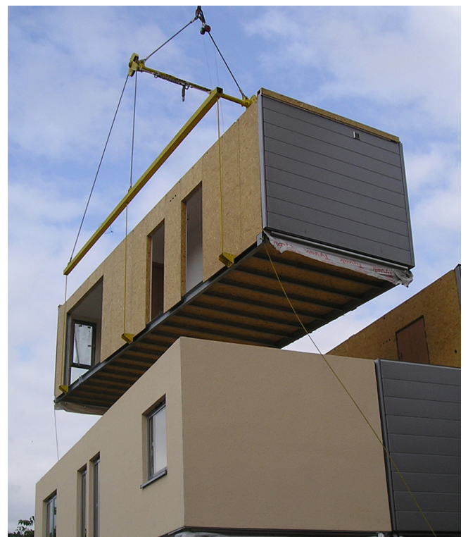
Fig.8 Installation of module with partially open sides
