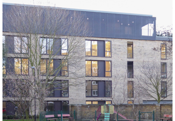
Fig.4 Residential building with apartments for rent, South London
