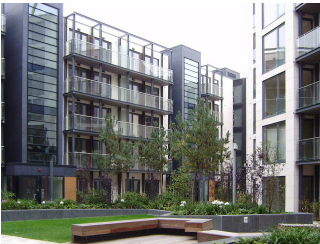
Fig.3 Courtyard view of modular residential buildings with large balconies, UK
