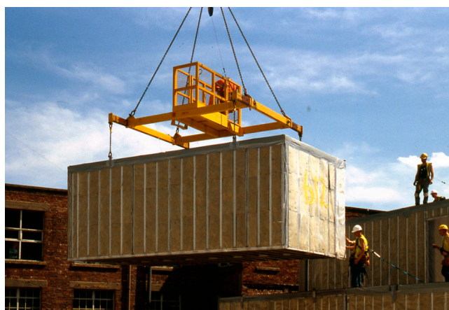
Fig.18 Installation of module from a protective cage
