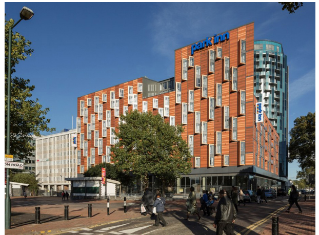
Рис.10 12-storey hotel in Wembley, North London
