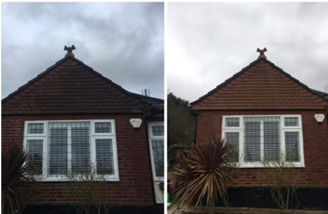
Tiling restored to its natural colour - Wickford, Essex
