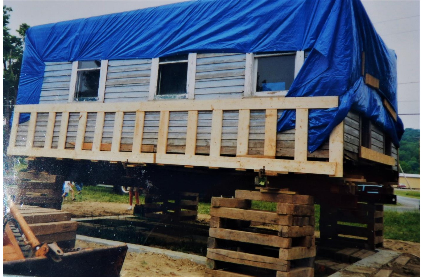
The school was placed in position waiting for the stone foundation to be put in place. The school would then be lowered into place.
