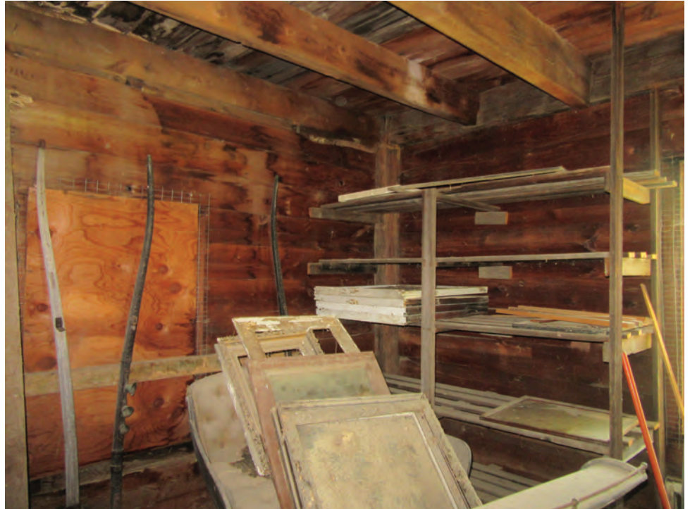
Figure 37 - Interior Grade Level View Towards South East Shop Corner – Salvaged Windows
