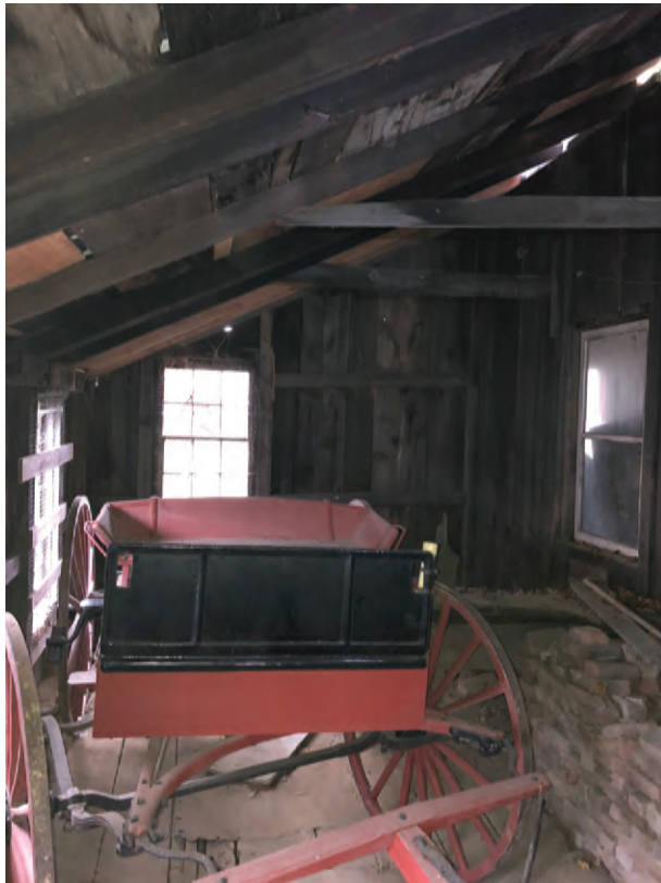
Figure 36 - Interior Grade Level View South – Lean-To
