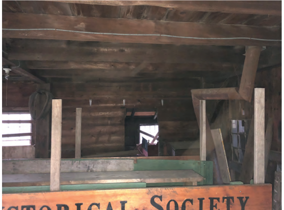
Figure 33 - Interior Grade Level – Entrance to Lean-To From Original Structure
