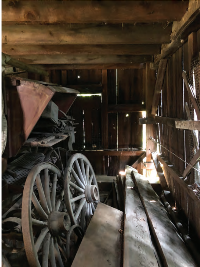
Figure 65 - Interior Grade Level View – Southeast Corner
