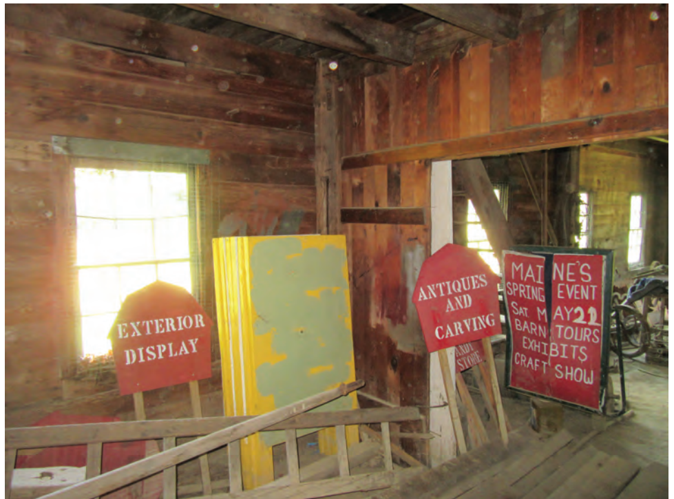
Figure 32 - Interior Grade Level View Towards North West Corner - Addition
