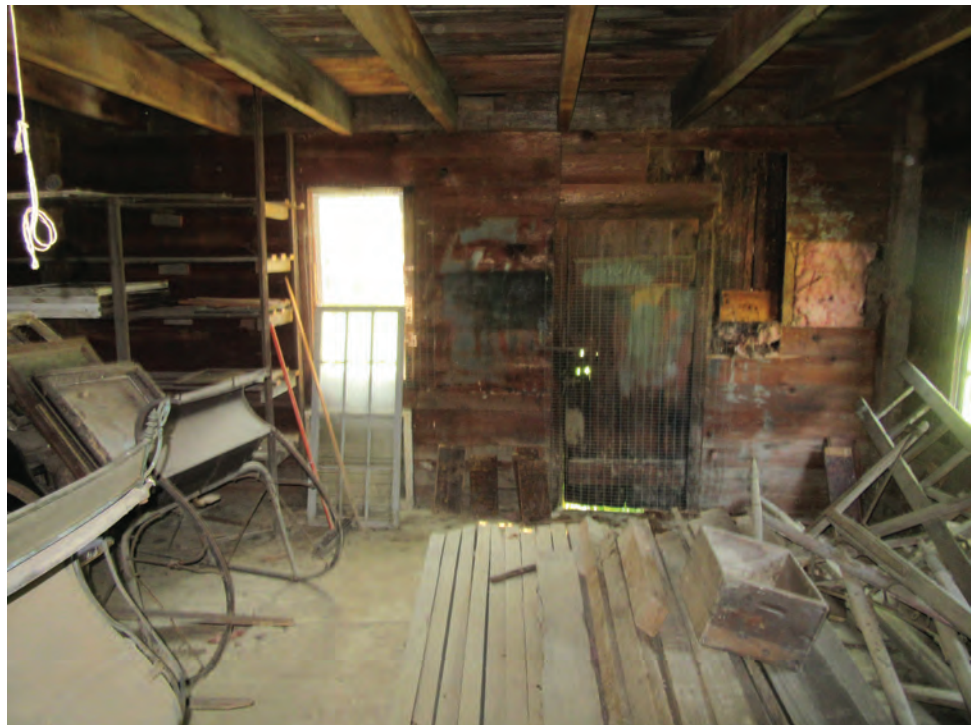
Figure 30 - Interior Grade Level View Towards South Wall - Addition
