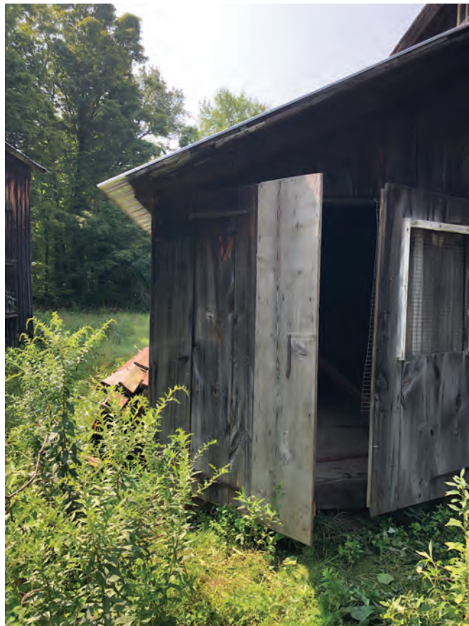
Figure 20 - North Elevation Lean-To
