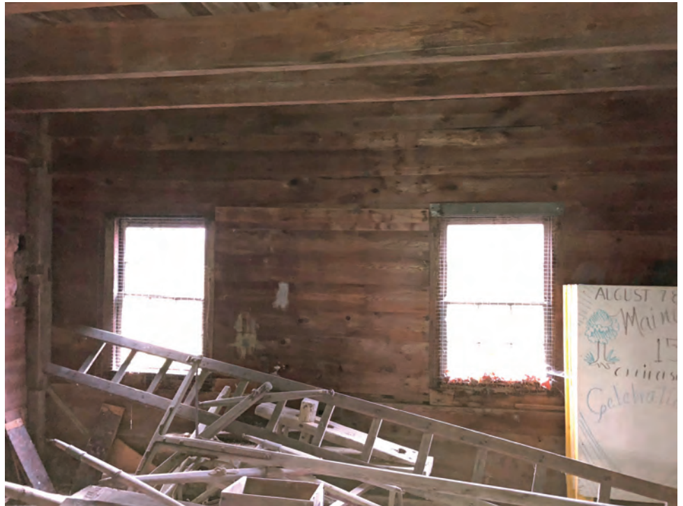
Figure 31 - Interior Grade Level View Towards West Wall - Addition
