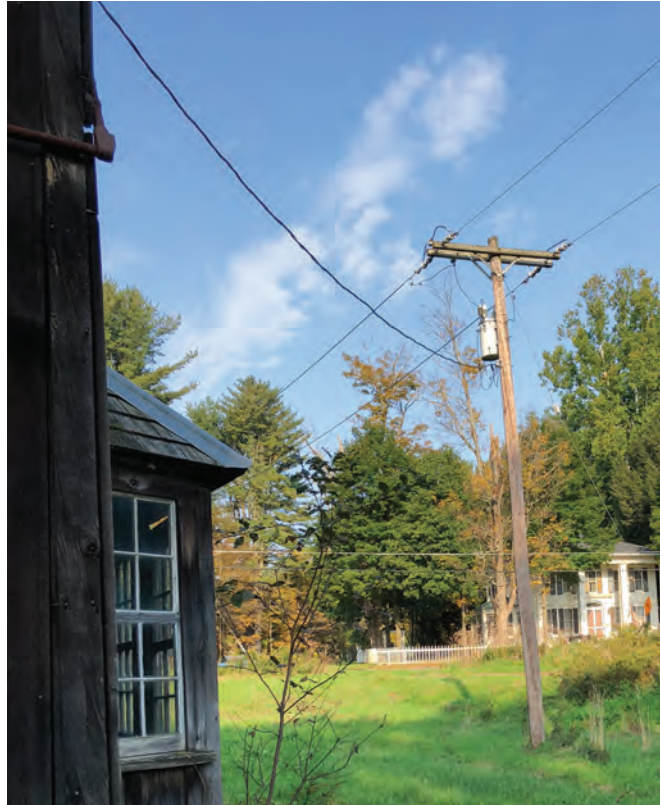
Figure 7 - Overhead Electric Service
