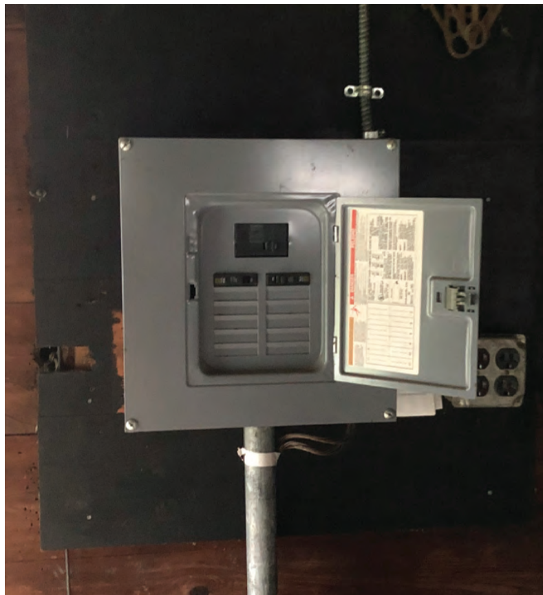
Figure 38 - Electrical Service Panel
