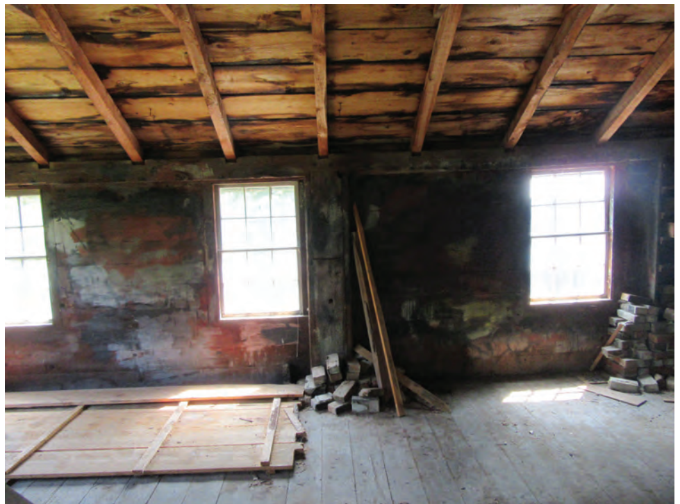
Figure 40 - Interior Second Level View East – Original Structure
