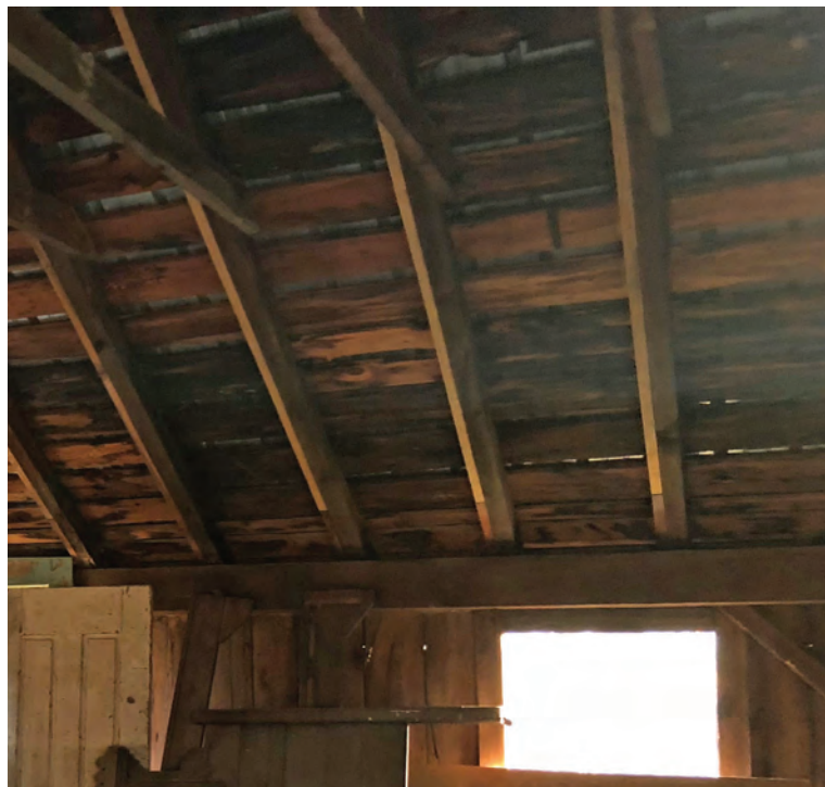
Figure 80 - Reinforcing at Wood Roof Framing
