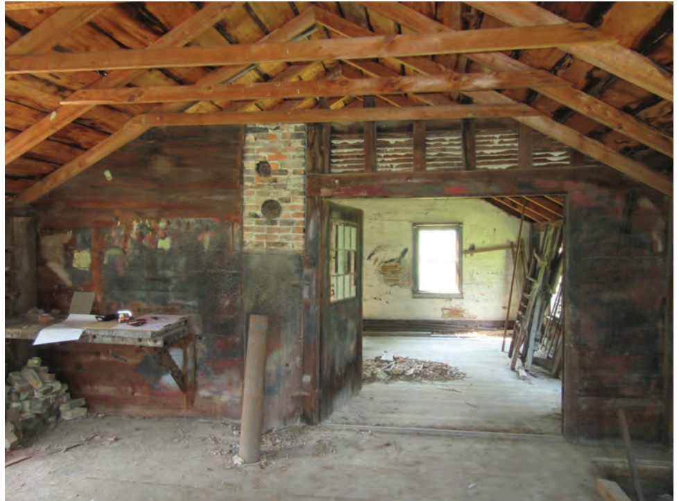
Figure 41 - Interior Second Level View South Towards Addition – Original Structure
