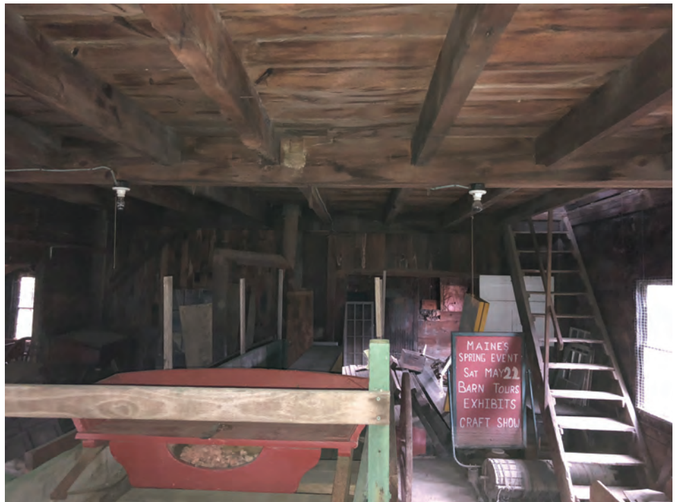
Figure 26 - Interior Grade Level View South – Original Structure- Opening to Addition in Center, Stairs to Second Level on Right
