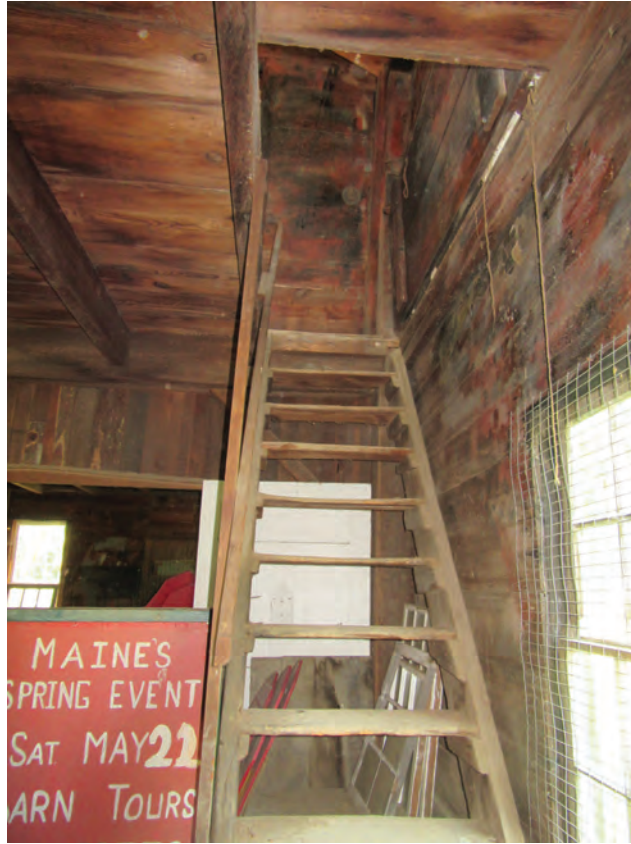
Figure 27 - Interior Grade Level View South –Stairs to Second Level
