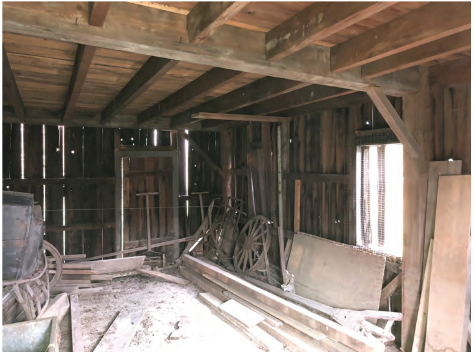
Figure 66 - Interior Grade Level View – Southwest Corner
