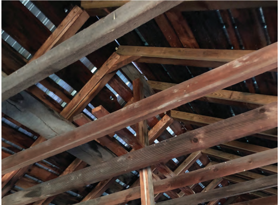
Figure 81 - Roof Framing and Intermediate Post
