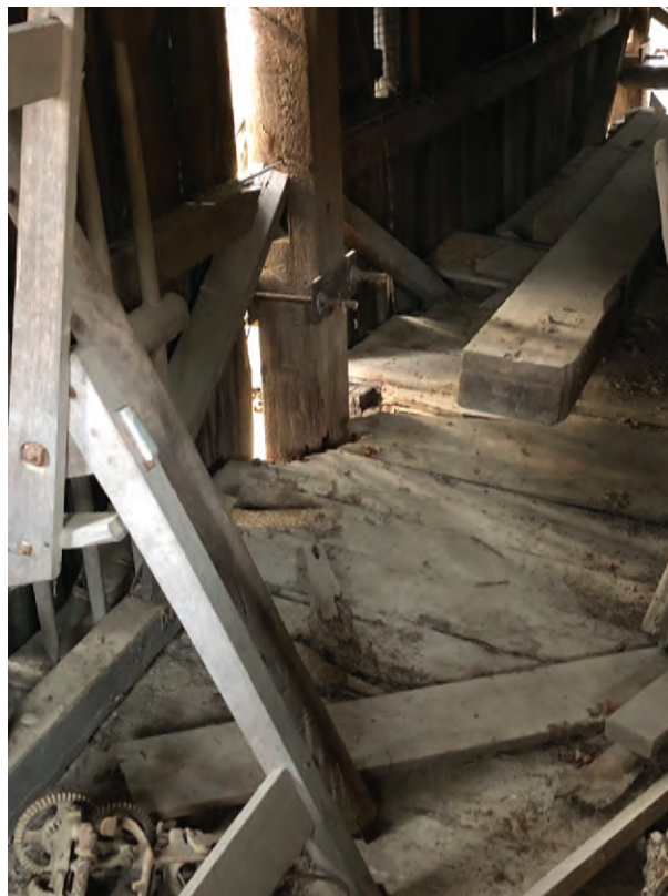
Figure 70 - Stabilization Measure at Missing Floor and Sill Beam Building Perimeter
