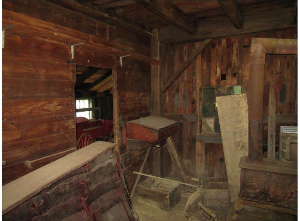
Figure 25 - Interior Grade Level View South West Corner – Original Structure – Entrance to Lean-To on left, Dividing Wall Between Addition on Right
