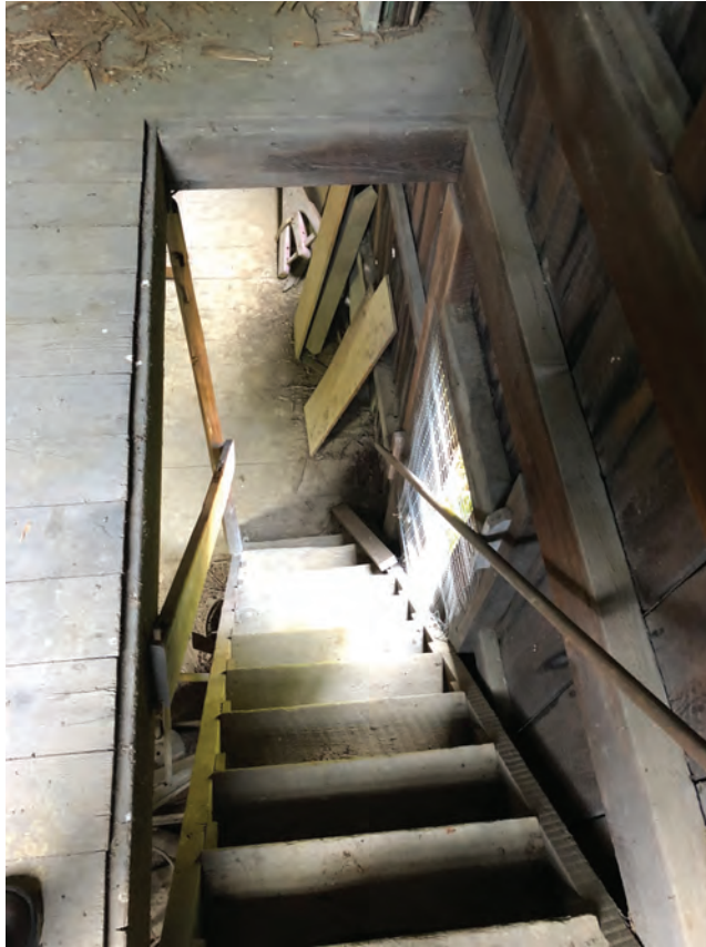
Figure 75 - Interior View – Second Level Looking Down Stairs
