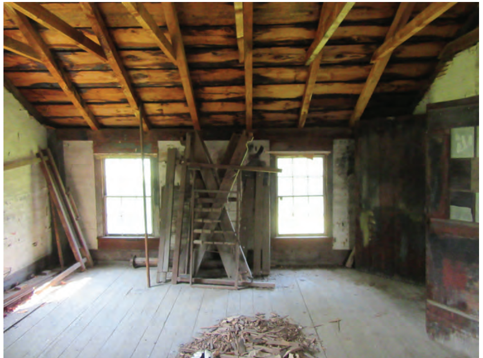
Figure 46 - Interior Second Level View West – Addition
