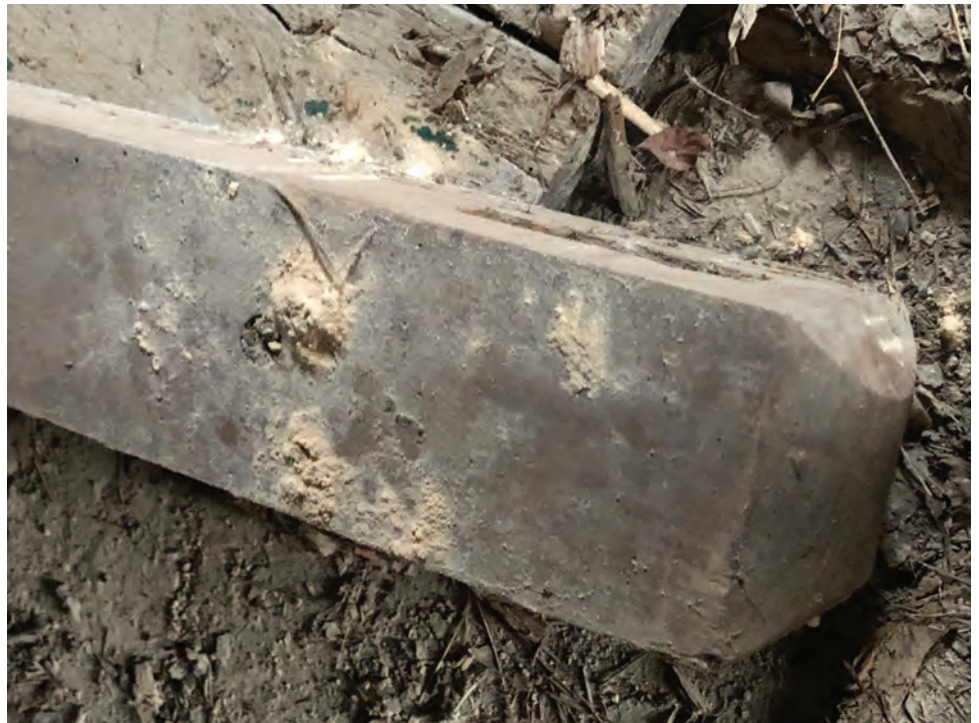
Figure 74 - Evidence of Powder Post Beetle Activity
