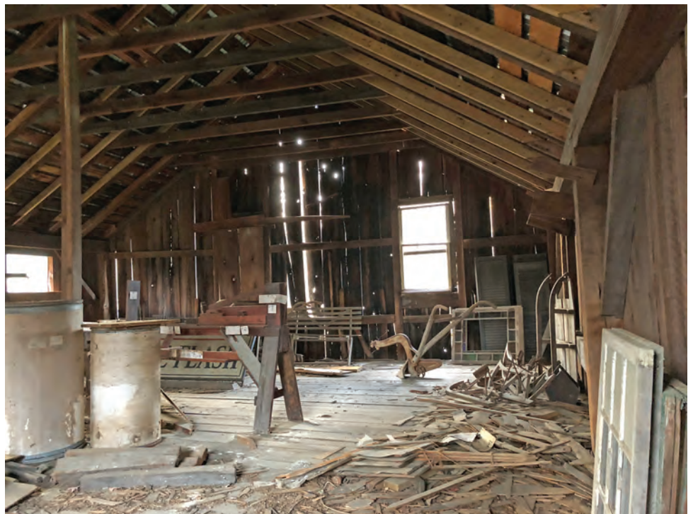
Figure 78 - Interior View Second Level – South Wall
