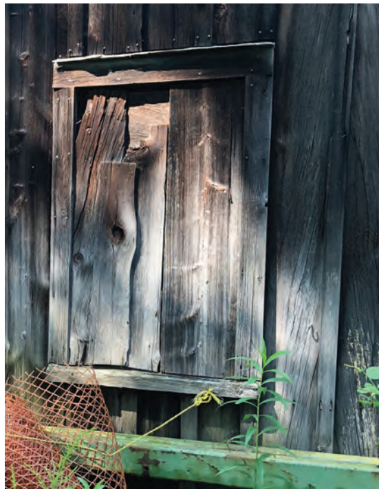
Figure 56 - Typical Boarded Finished Window
