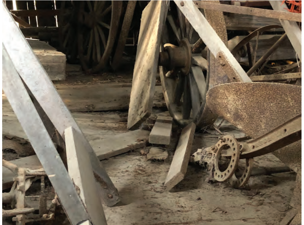
Figure 73 - Sagging Subfloor at Interior Floor Span
