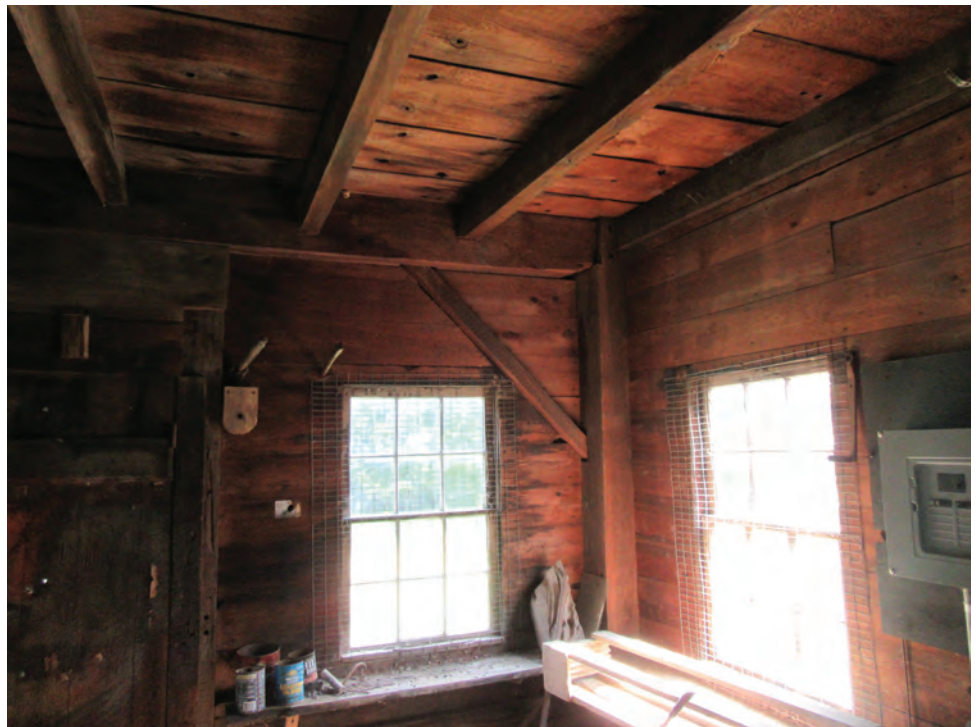
Figure 24 - Interior Grade Level View North West Corner - Original Structure
