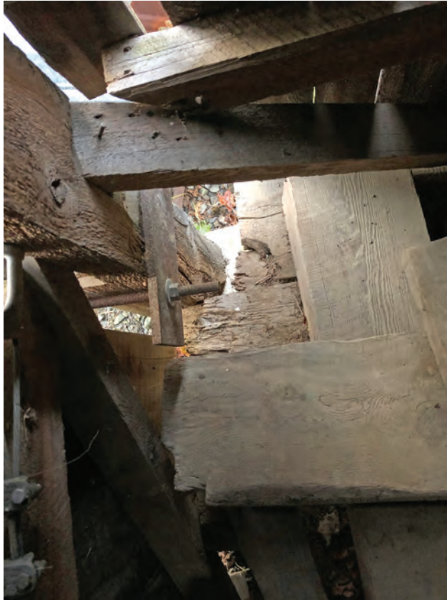
Figure 71 - Stabilization Measure at Missing Floor and Sill Beam Building Perimeter
