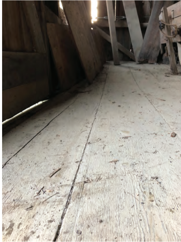
Figure 69 - Floor Level Drop – View From North Center Towards Northeast Corner
