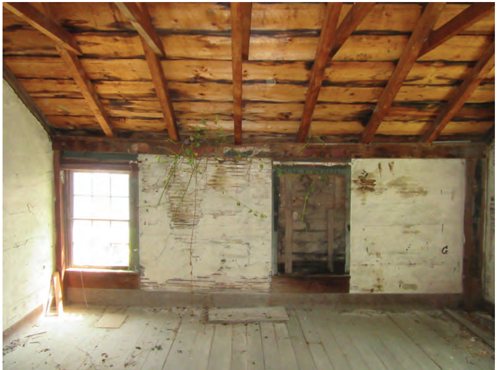
Figure 44 - Interior Second Level View East – Addition
