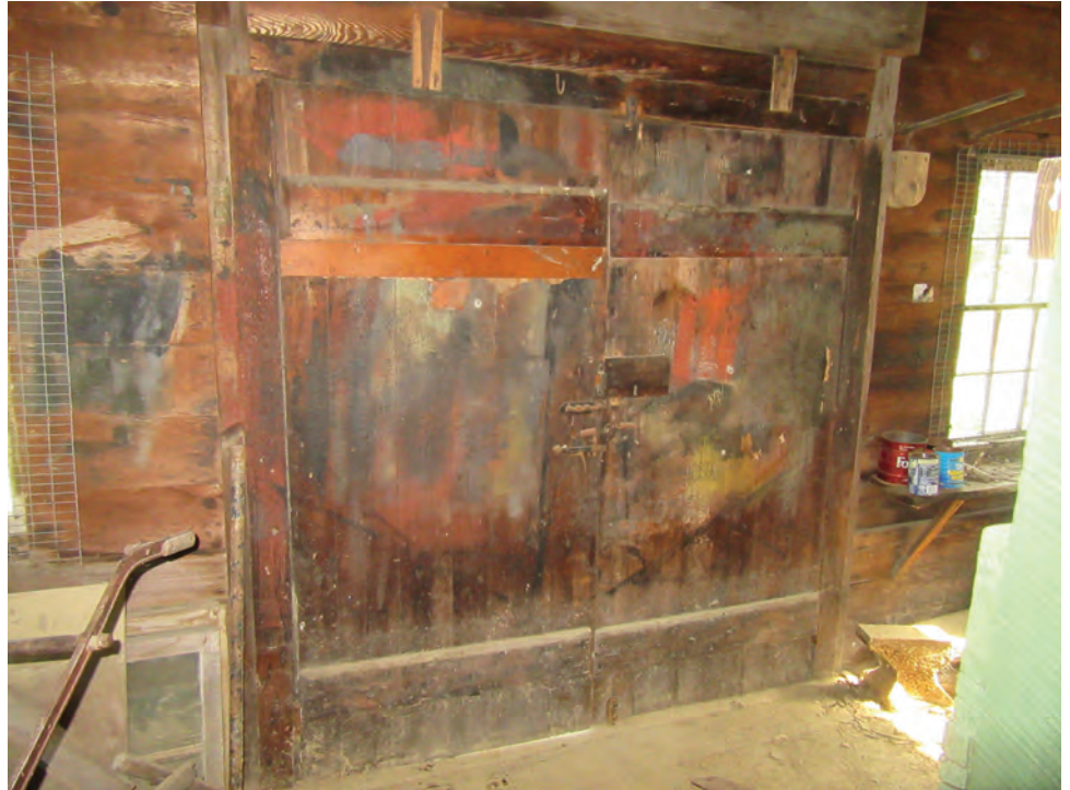
Figure 19 - Grade Level Shop Doors - Interior
