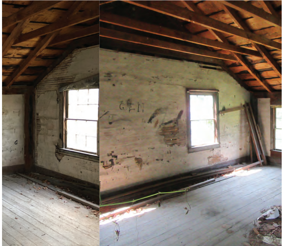
Figure 45 - Interior Second Level View South – Addition
