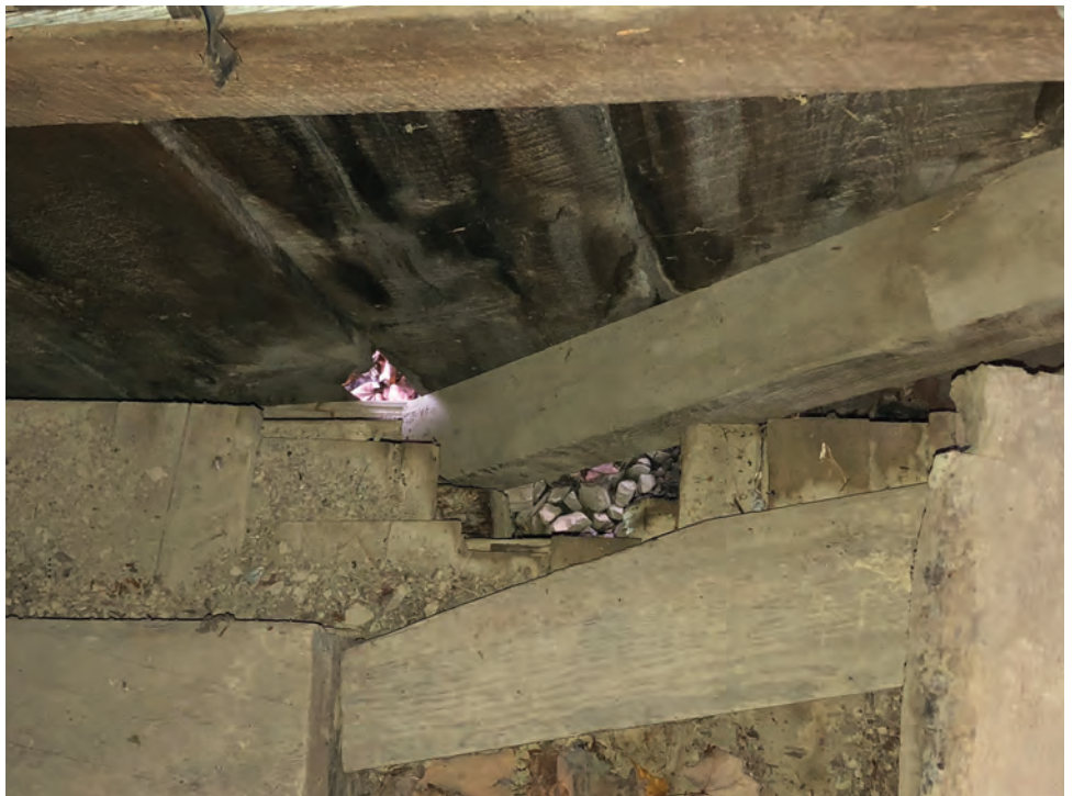
Figure 72 - Stabilization Measure at Missing Floor and Sill Beam Building Perimeter
