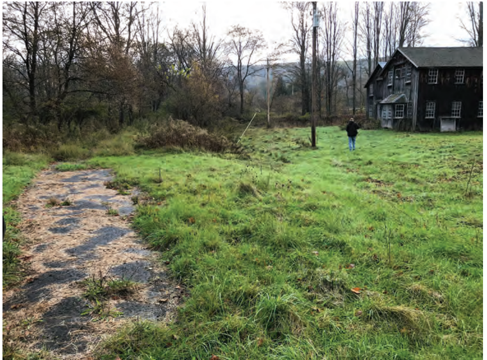
Figure 6 - Abandoned Road Bed With Partial Macadam Paving Visible
