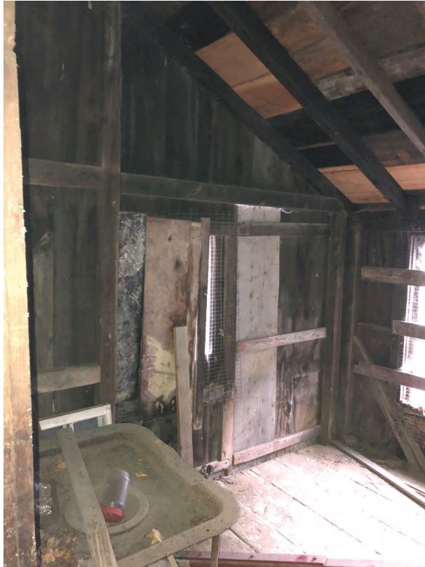
Figure 35 - Interior Grade Level View North – Lean-To
