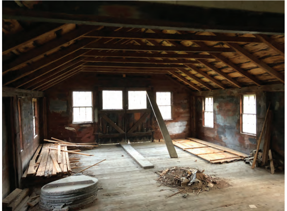
Figure 39 - Interior Second Level View North From Top of Stairs – Original Structure
