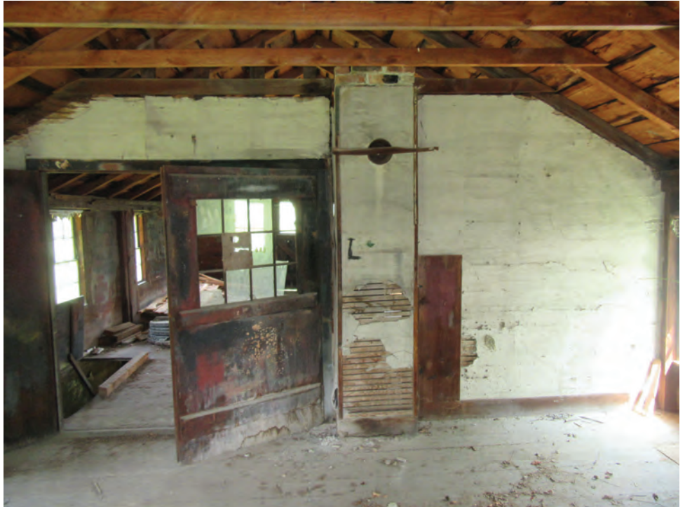
Figure 43 - Interior Second Level View North Towards Original Structure – Addition
