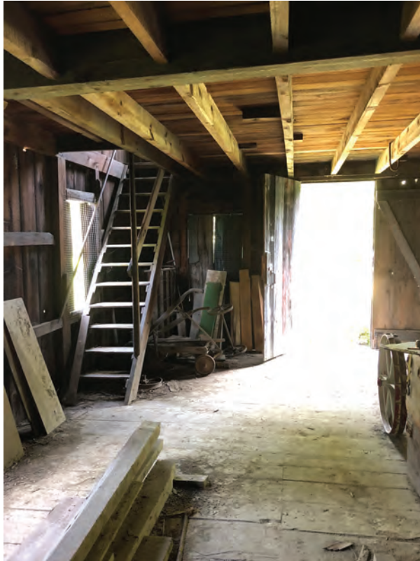
Figure 67 - Interior Grade Level View – North Entrance Doors and Stair to Second Level
