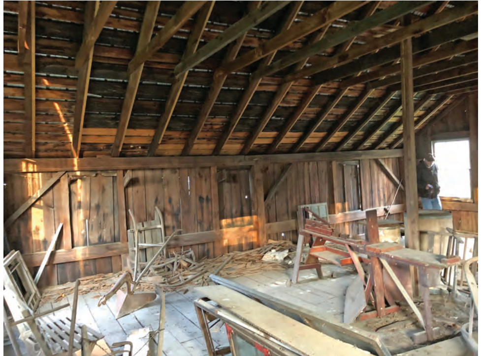
Figure 79 - Interior View Second Level – West Wall
