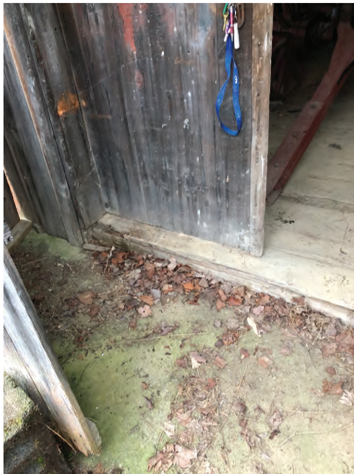
Figure 22 - Bayed doors entrance with step up
