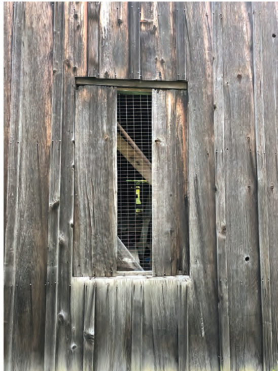
Figure 62 - Typical Boarded Unfinished Window Opening
