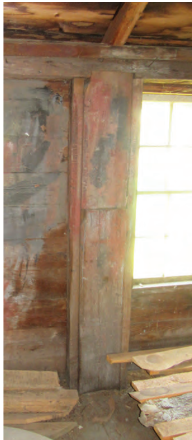
Figure 42 - Second Level Post With Visible Splice – Original Structure
