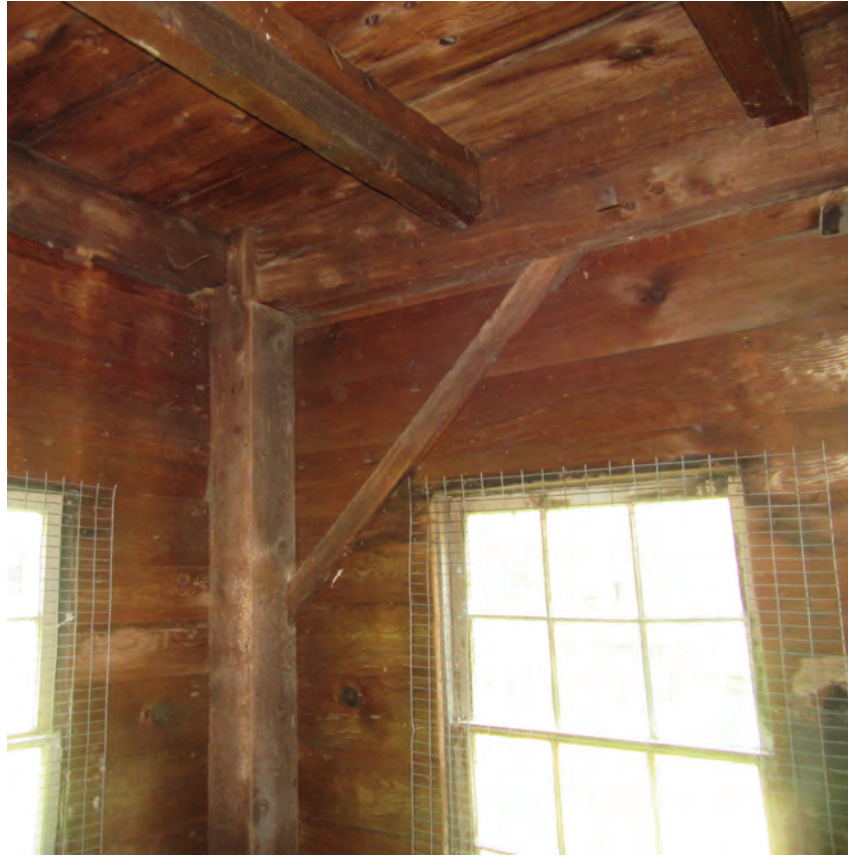
Figure 23 - Typical Shop Interior Framing Components
