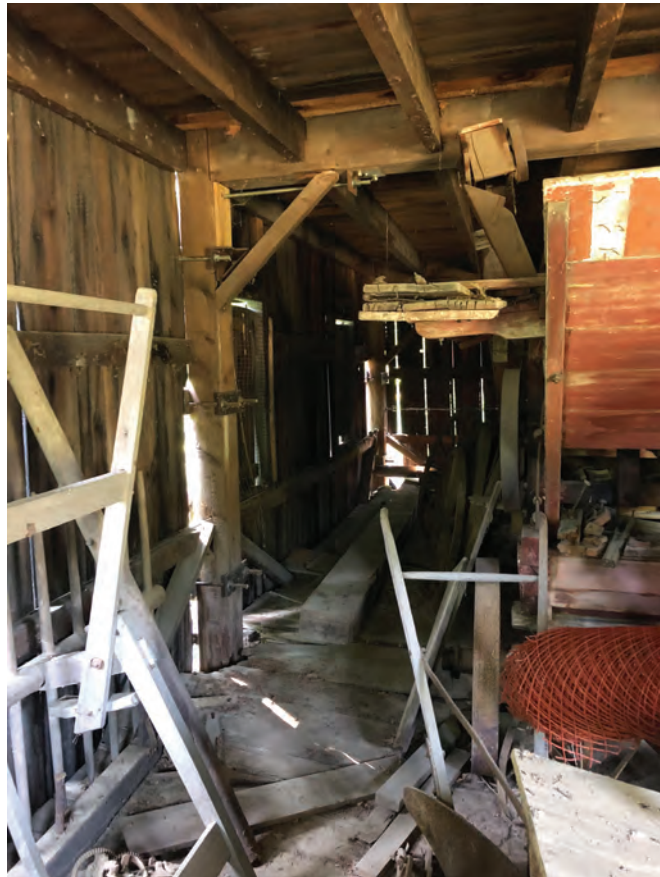
Figure 64 - Interior Grade Level View – East Wall
