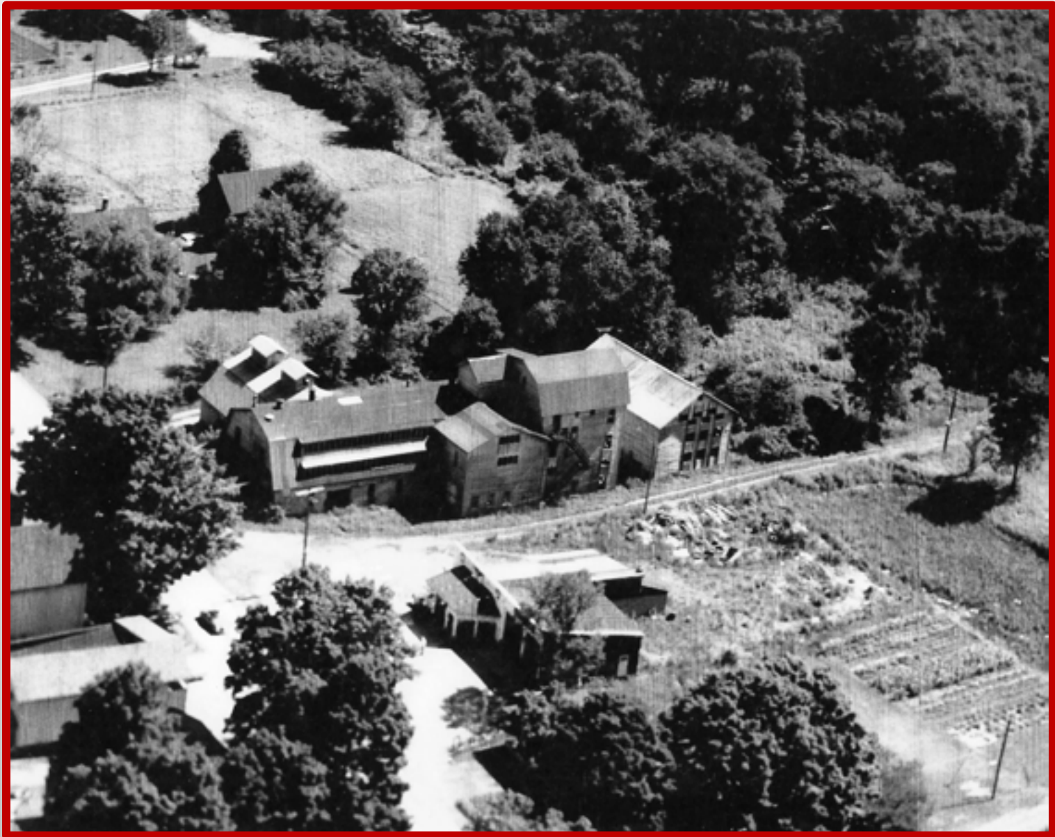
Dairyman's League Cooperative Association's Maine plant before 1964 when it burned down along with 5000 hens.
