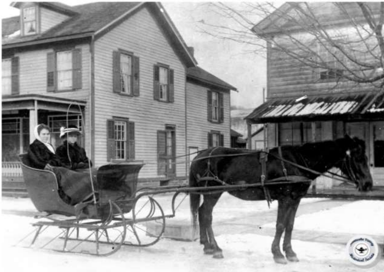
1908- The preferred mode of transportation in winter were sleighs and cutters—light sleighs. Note the high, curved dash in front which deflected snow and ice. The cut rock at the sidewalk was used for getting into sleighs.
