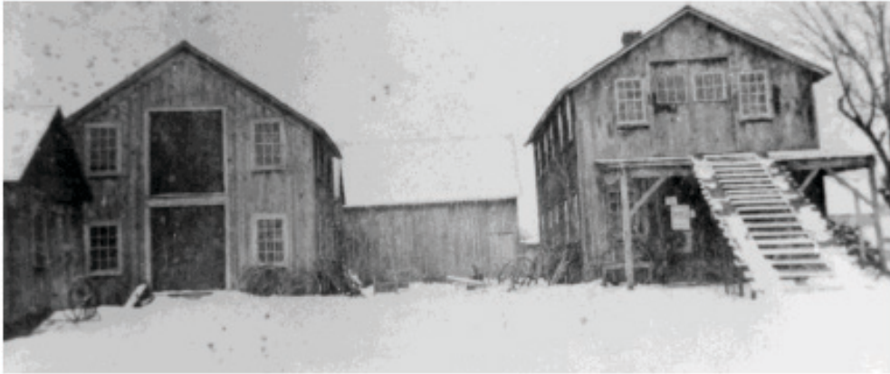
1899 image of the Norton buildings, looking south
