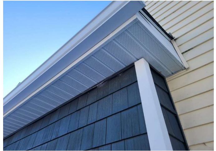
Soffit and fascia at roof eave
