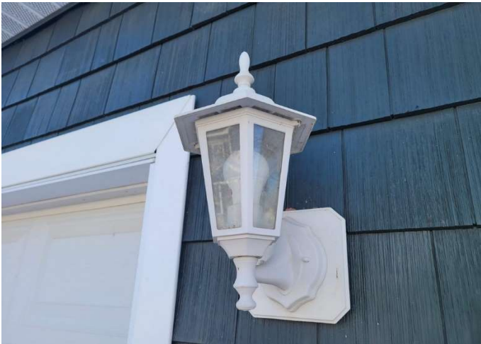
Typical sconce at front façade
