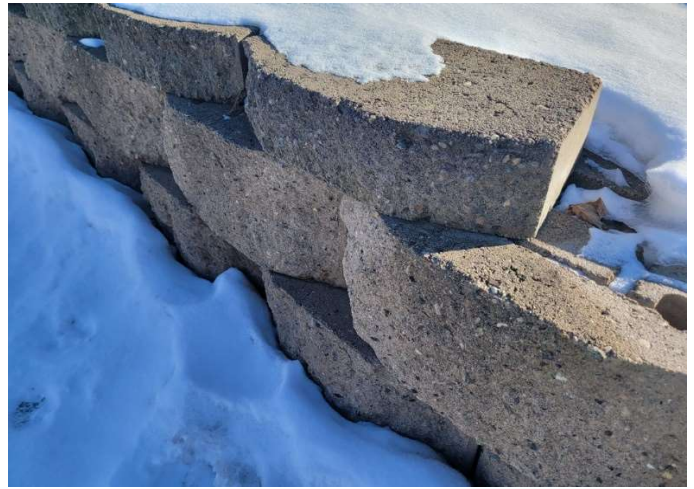
Segmental masonry unit retaining wall
