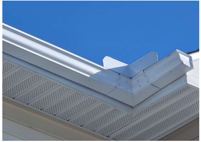
Gutter at eave with diverter
