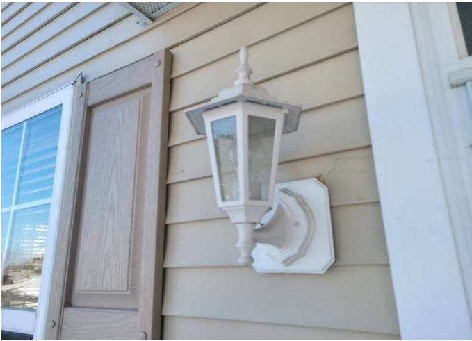
Sconce near entry door
