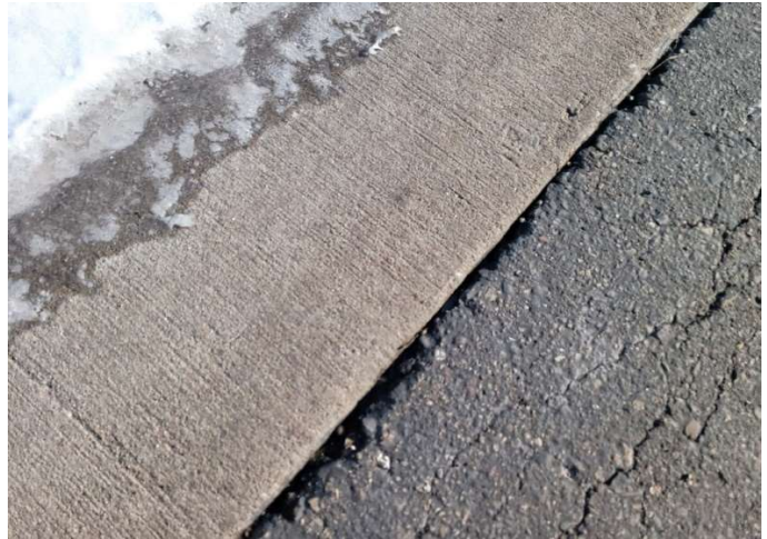
Gutter between drive and concrete driveway
