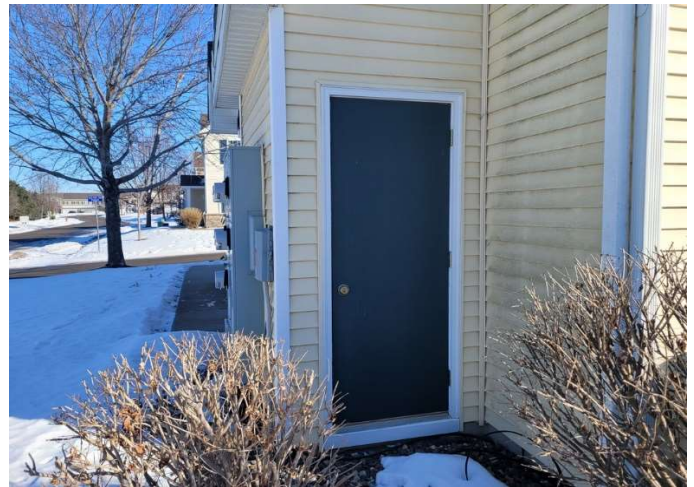
Overview of metal utility door
