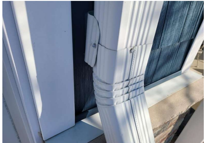
Connected downspout sections
