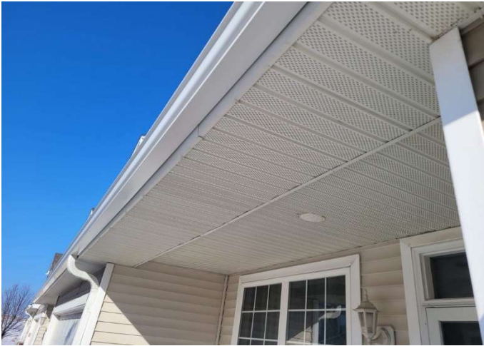
Soffit at covered entry
