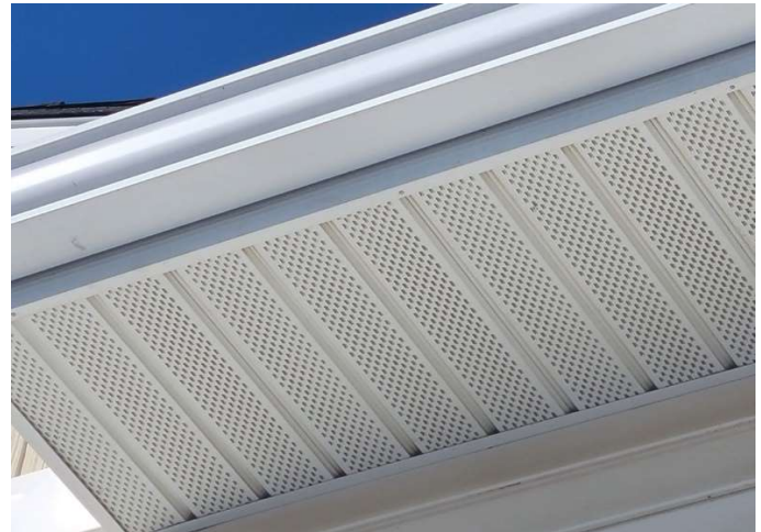
Soffit and fascia at roof eave
