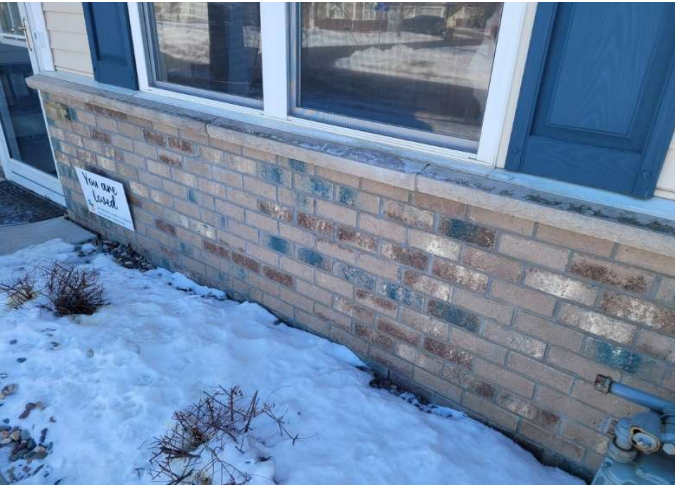
Brick masonry overview
