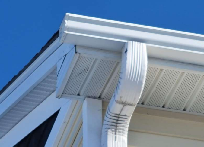
Gutter to downspout connection at eave
