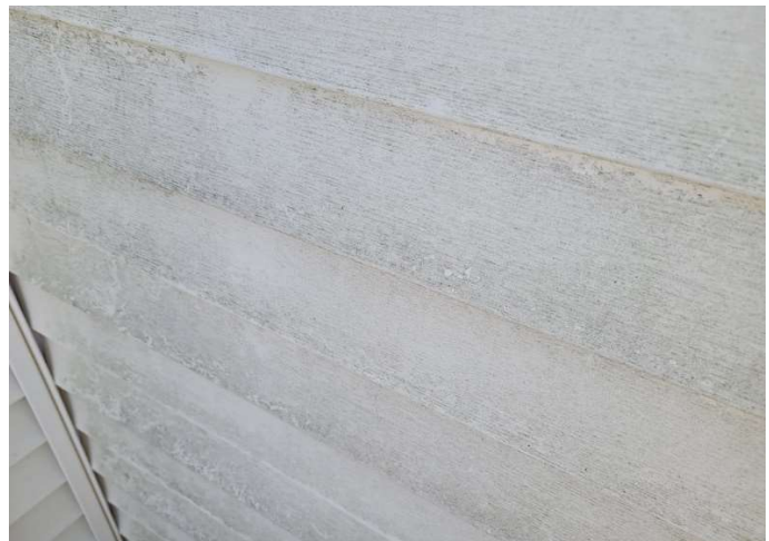
Siding with dirt and organic growth (fund power washing and cleaning through operating budget)
