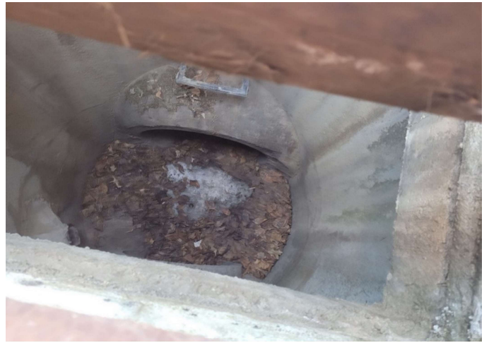
Catch basin interior
