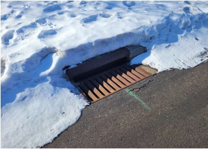
Overview of catch basin
