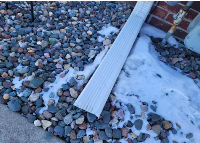
Downspout extension at grade
