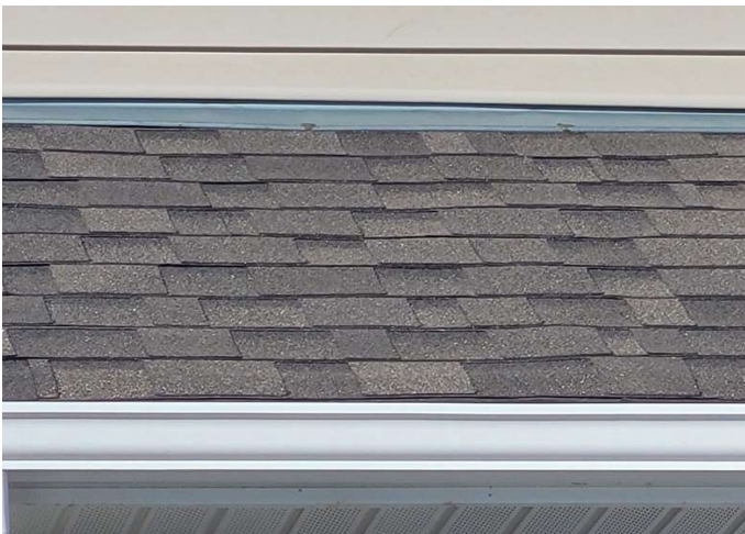
Shingles at lower roof level
