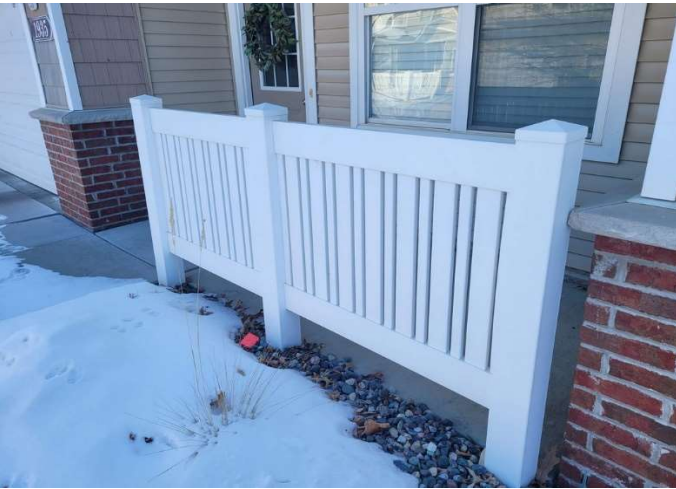
Vinyl fencing at front patio
