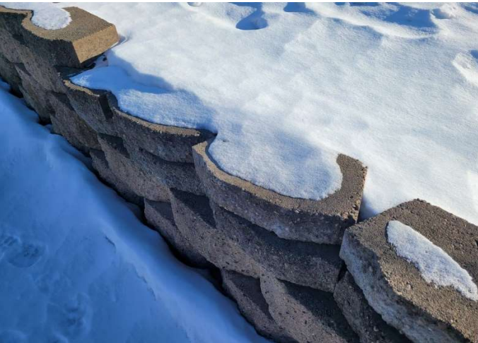
Segmental masonry unit retaining wall
