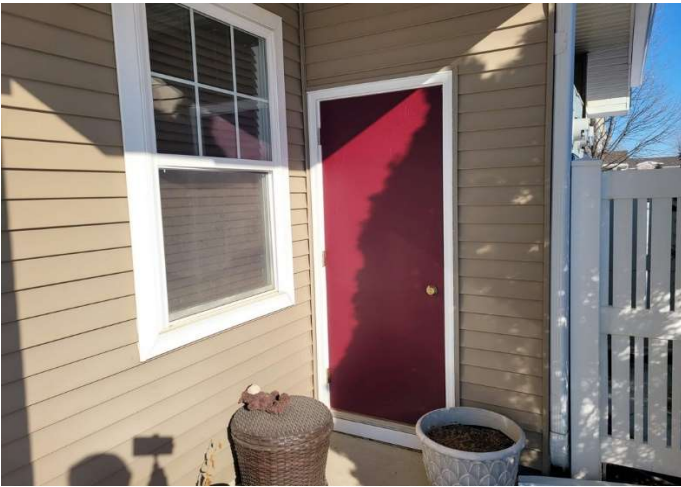
Overview of metal utility door
