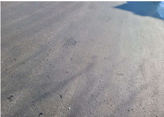
Section of smooth pavement with few cracks
