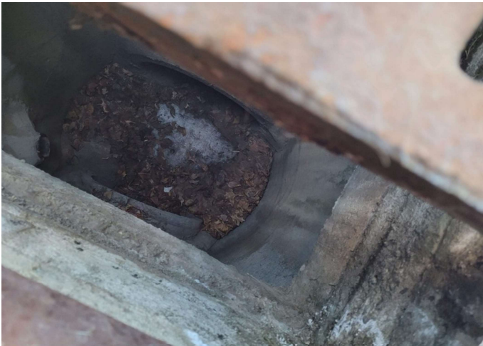
Catch basin interior
