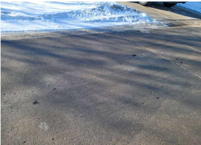
Section of smooth pavement with few cracks
