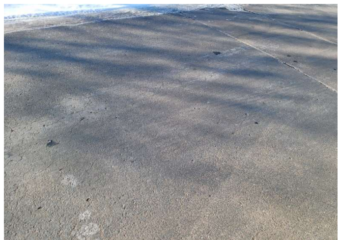
Section of smooth pavement with few cracks
