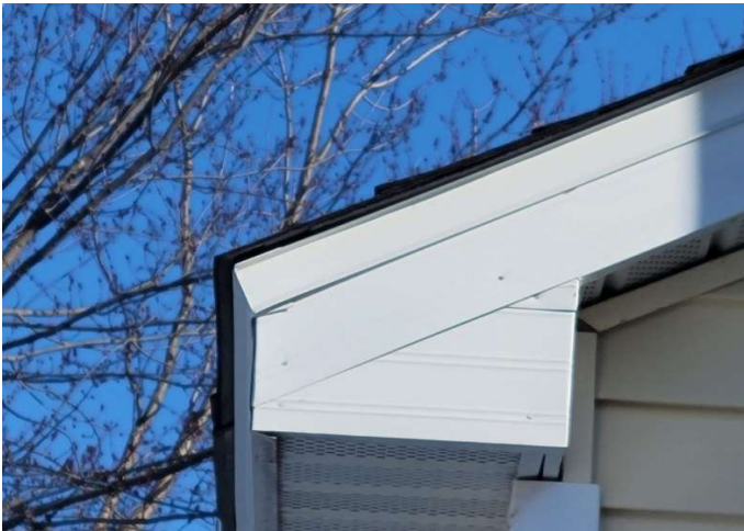
Fascia trim at eave
