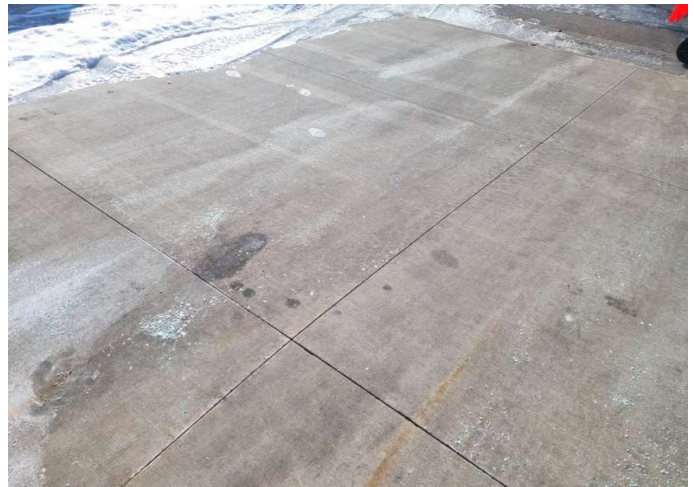
Concrete driveway installed in 2017
