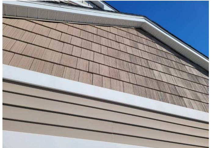
Vinyl siding above garage door
