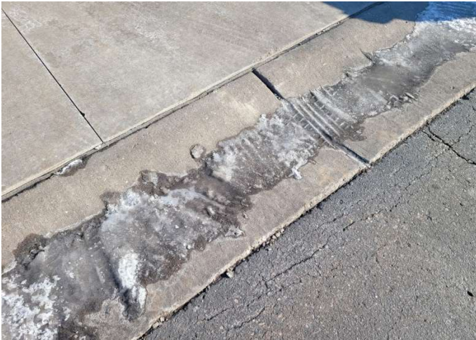
Overview of concrete curb and gutter
