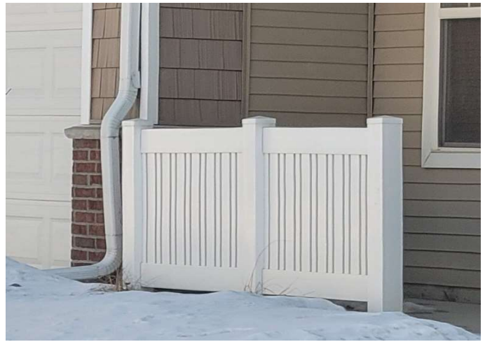
Vinyl fencing at front patio
