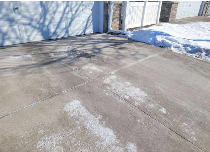
Concrete driveway installed in 2017
