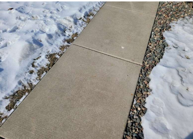
Concrete sidewalk connecting driveway to unit entry area
