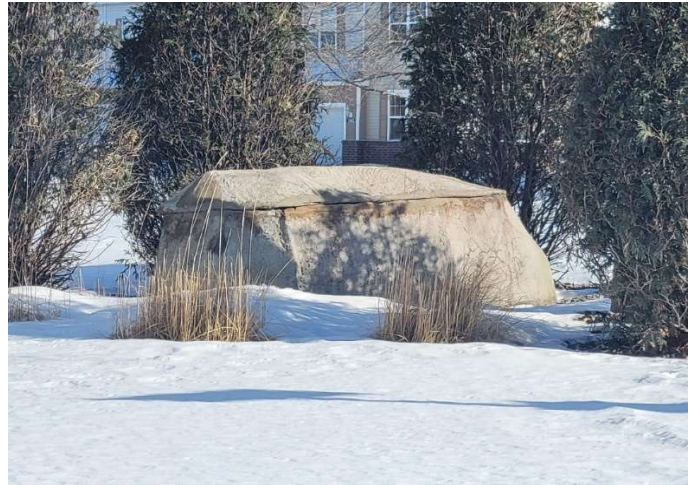
Irrigation valve location
