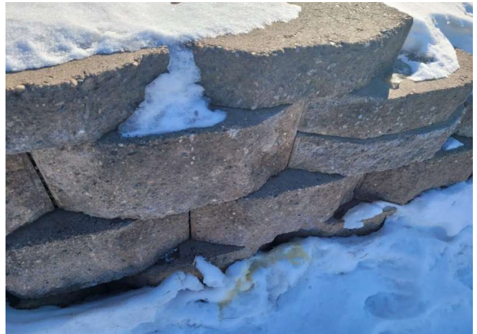
Segmental blocks and caps at retaining wall
