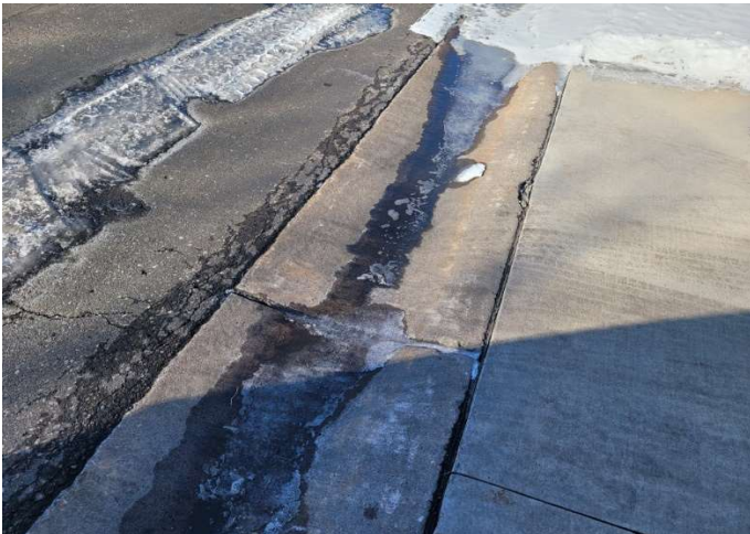
Gutter between drive and concrete driveway
