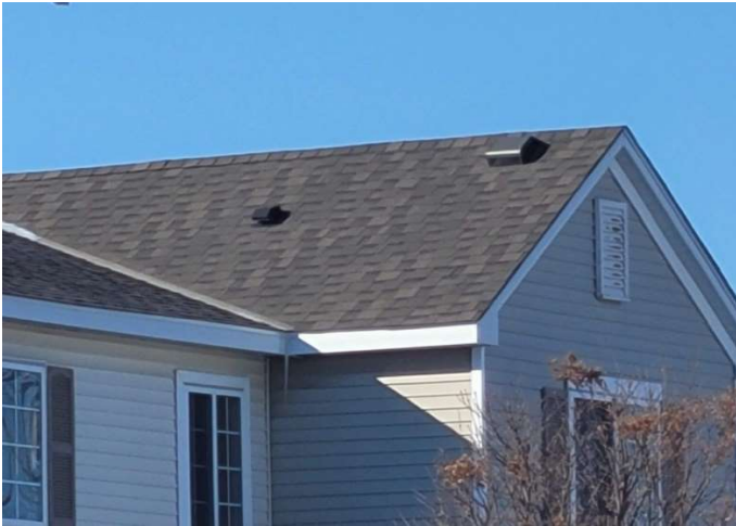
Overview of asphalt shingle roof
