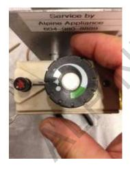
Position two is to turn the dial to the spark "star" to ready for lighting.
