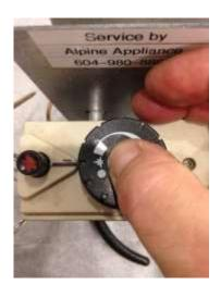
We start gas to flow to the pilot by depressing the button in the "spark" position down.
