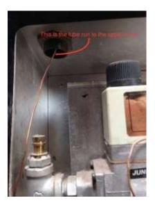
This thermo-sensor connected to the gas valve must be removed before the burner can be removed from the burner compartment.
