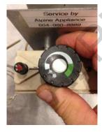
You can them continue to turn the control dial counterclockwise, so the indicator line (black line) is in line with the start of the green on the dial. In some instances, a venting draft is not established in the AGA and the flame on the main burner will blow itself out. Once the main burner is a light, look though the sight glass to ensure the flame is not
